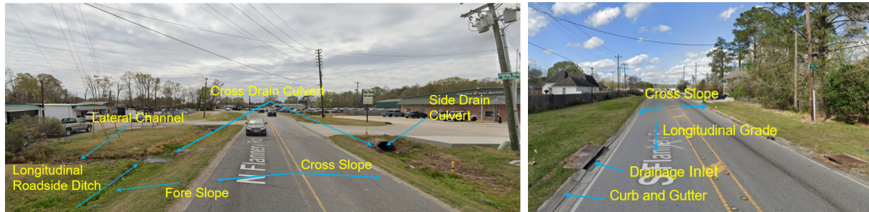
Figure 2. Pavement drainage system
