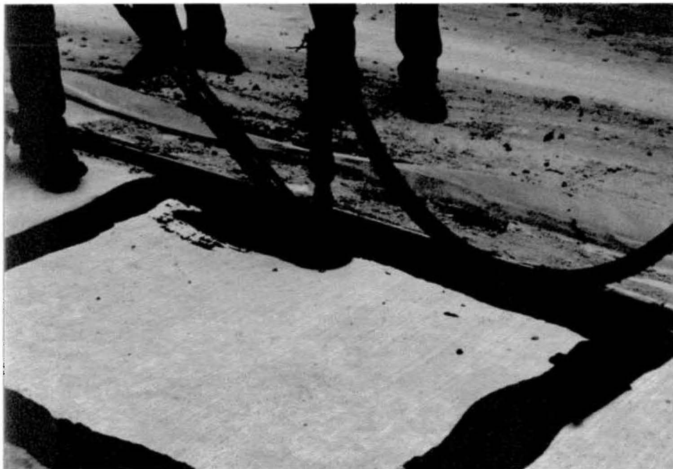
4. Installation of fiber-asphalt Sami.
