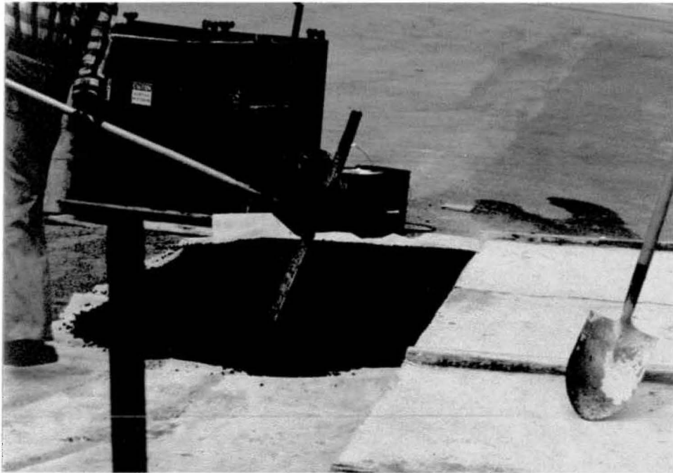
5. Paving for additional samples of overlay over flexible sections.
