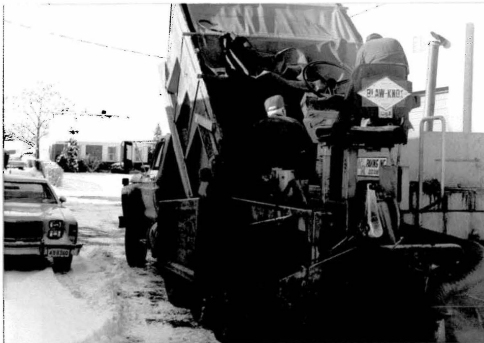
Photo 5. Paver being loaded for placement of overlay.
