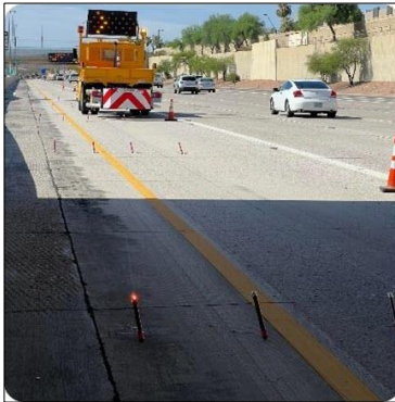
Figure 11. Typical Sampling Operations: HOV Closure
