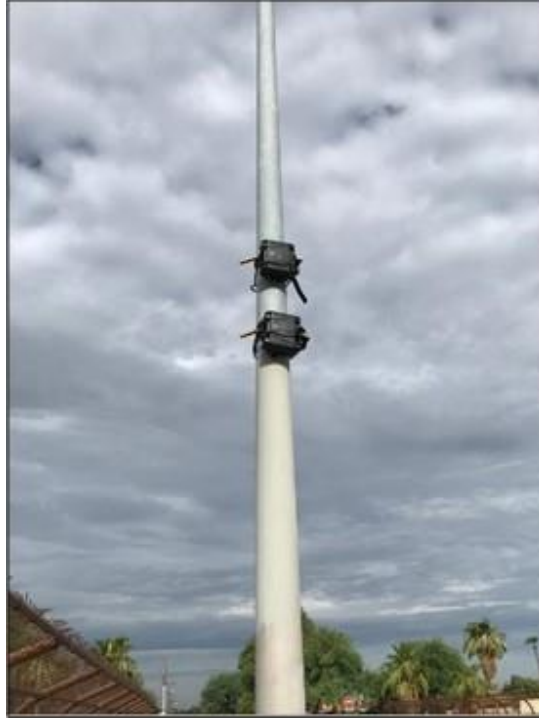
Figure 32. Setting Up Traffic Control at the Victory Drive Site and Traffic Counters Installed on a Pole
