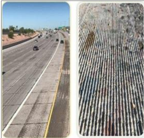
Figure 2. An Overview of a Pavement Surface after Diamond Grinding
