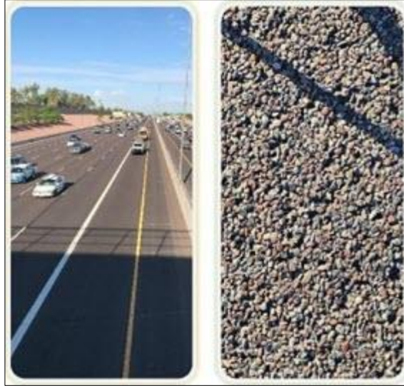
Figure 1. An Overview of Rubberized Asphalt Surface
