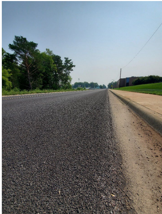
Fog-sealed Chip Seal in Curb and Gutter Section
