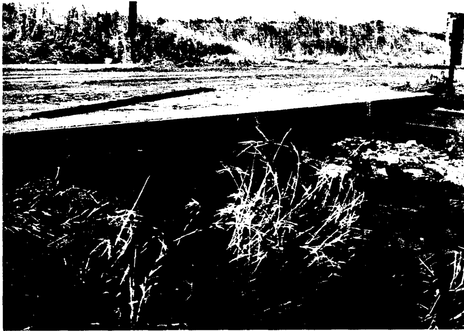
FIG. 4 SIMPLE LOW WATER BRIDGE
