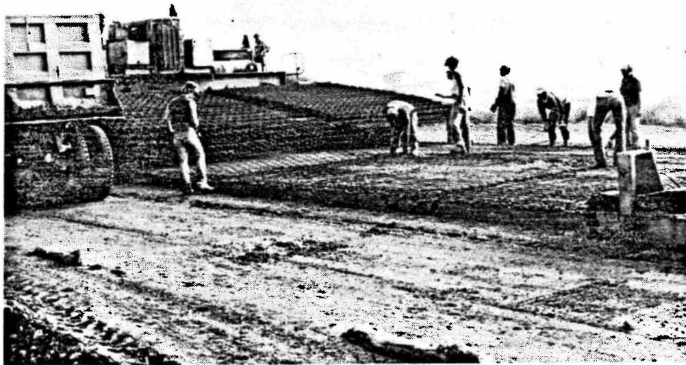
Figure 26. Overlap of steel-reinforcing mesh placed between concrete layers.
