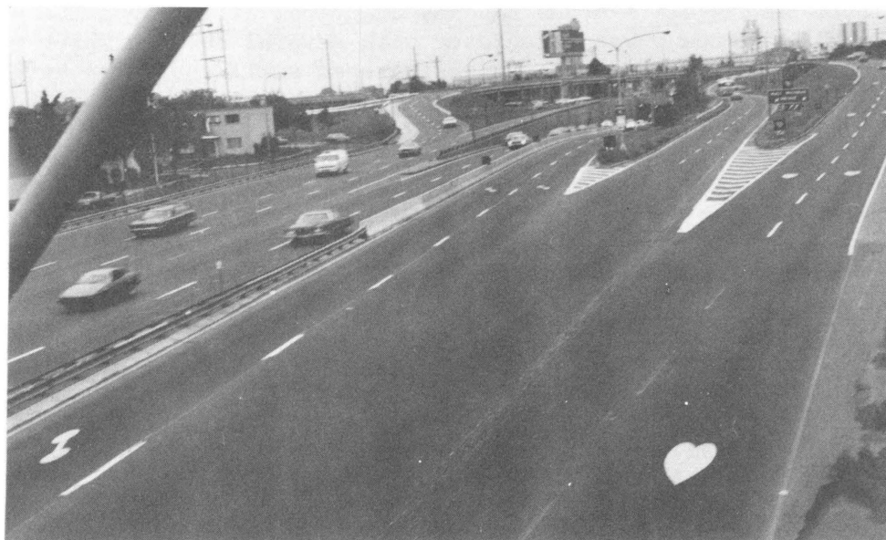
Figure 11. System E Pavement Symbols
