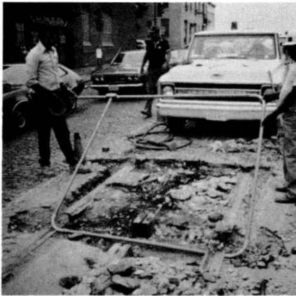
Figure 36. Enclosed Loop Configuration
