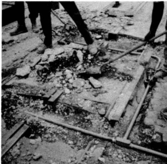
Figure 37. Enclosed Loop Installation
