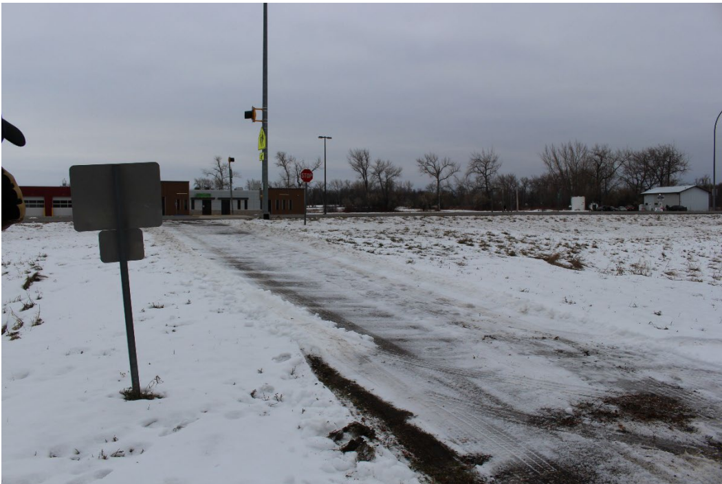
Figure 5.4 Slippery sidewalk conditions
