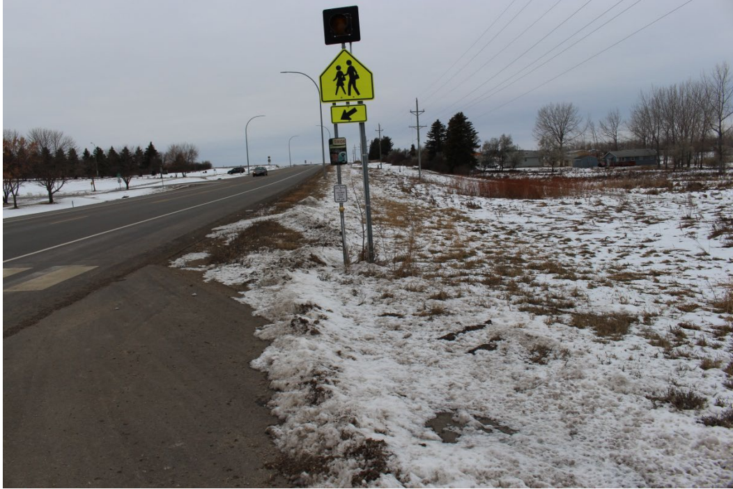
Figure 5.11 Another location with missing landing for pedestrian push button
