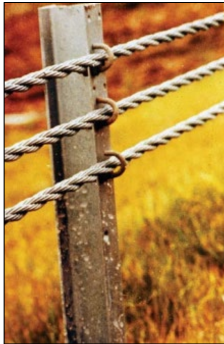
Figure 104. Photograph. Example three-strand cable. (59)
