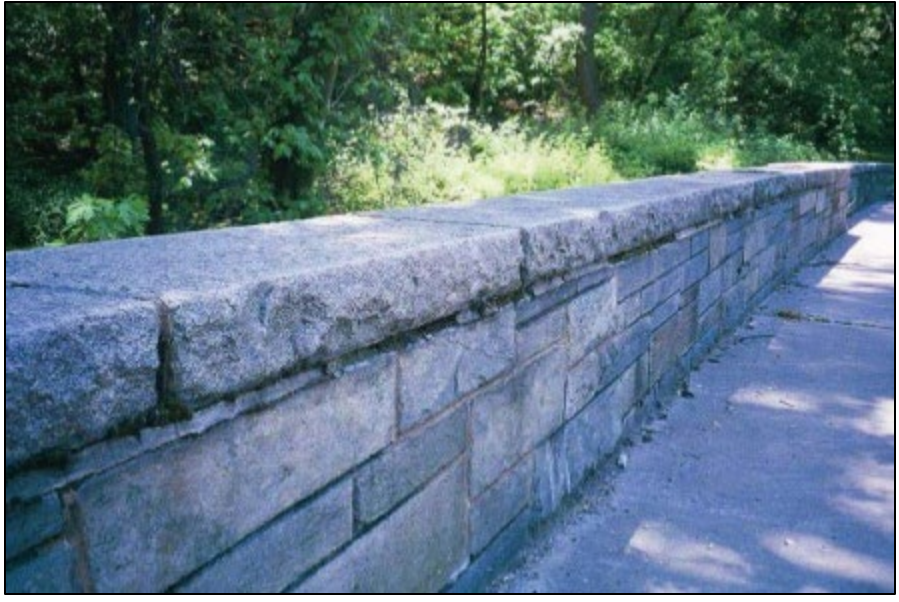
Figure 67. Photograph. Example precast concrete guardwall. (59)
