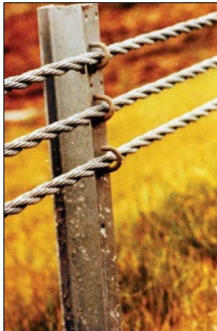
Figure 73. Photograph. Example high-tension cable. (59)
