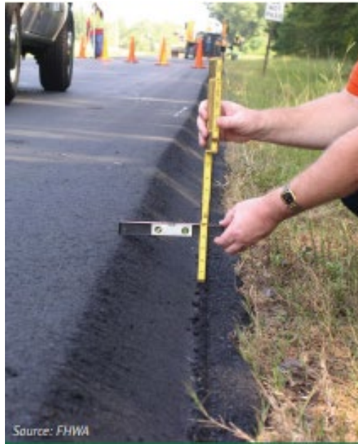
Figure 78. Photograph. SafetyEdge SM example. (68)
