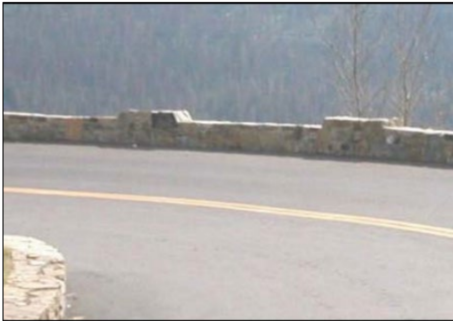
Figure 77. Photograph. Example random rubble cavity wall. (59)
