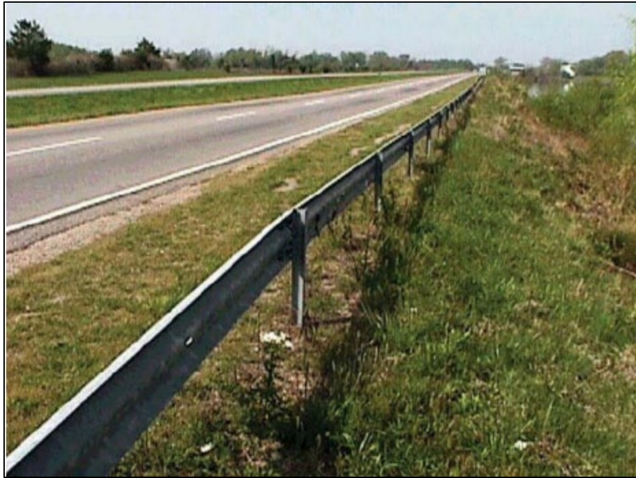
Figure 75. Photograph. Example weak post w-beam. (59)
