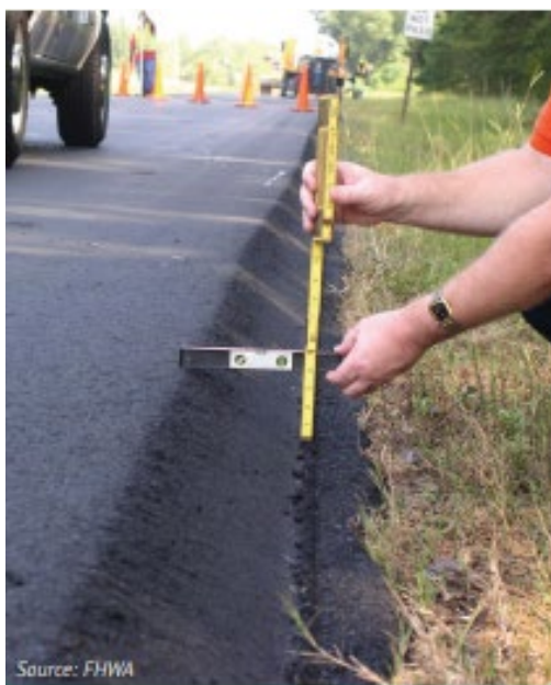
Figure 109. Photograph. SafetyEdge SM example. (68)
