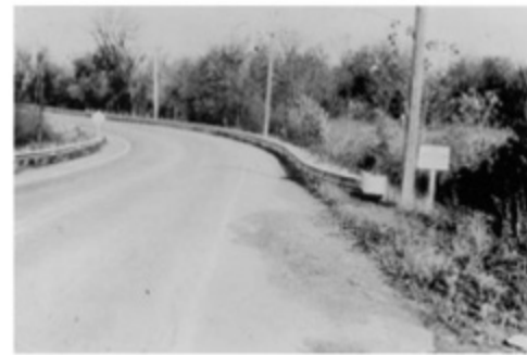
Typical Roadway with Roadside Hazard Rating Equal to 4.
