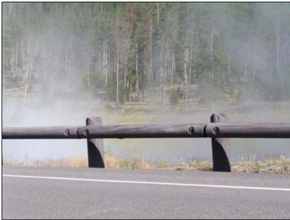
Figure 75. Photograph. Example weak post w-beam. (59)
