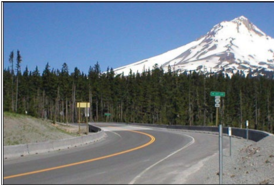
Figure 66. Photograph. Example concrete safety shape. (59)
