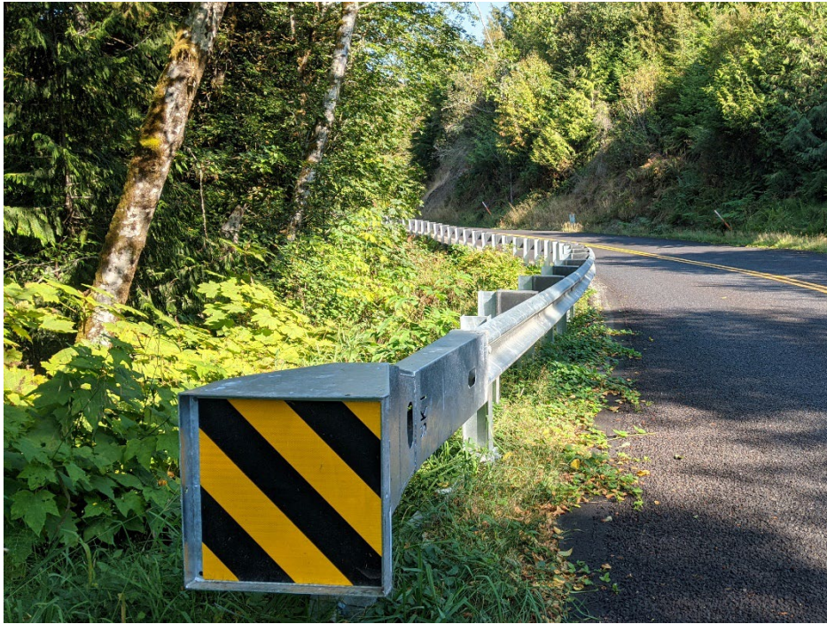
Figure 45. Photograph. Sight distance issue related to vegetation on the inside of a horizontal curve.
