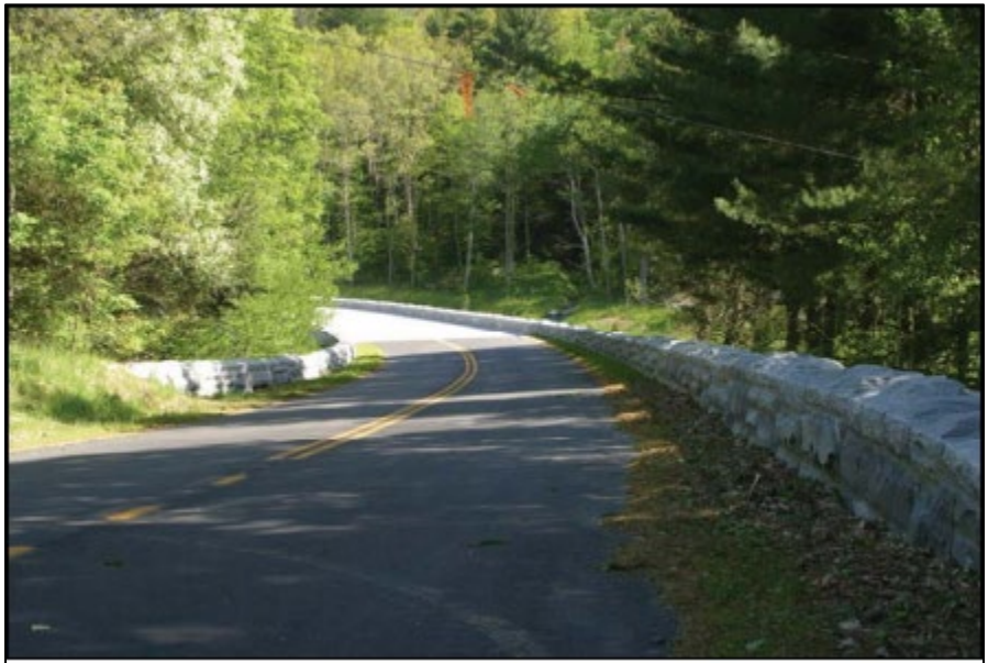
Figure 67. Photograph. Example precast concrete guardwall. (59)
