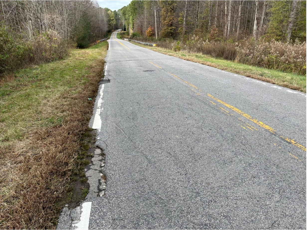
Figure 39. Photograph. Example of potholes and pavement edge deterioration.
