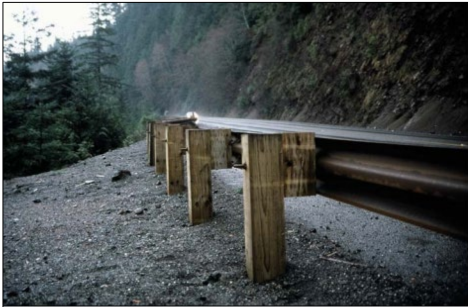
Figure 100. Photograph. Example box beam. (59)
