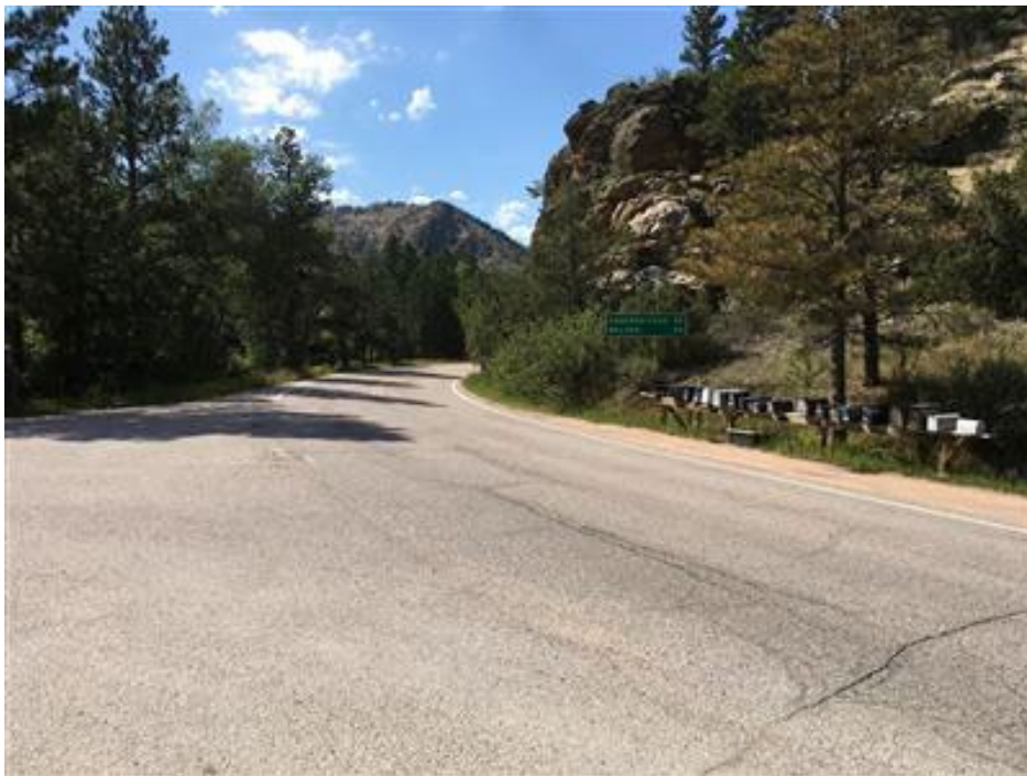
Figure 45. Photograph. Sight distance issue related to vegetation on the inside of a horizontal curve.
