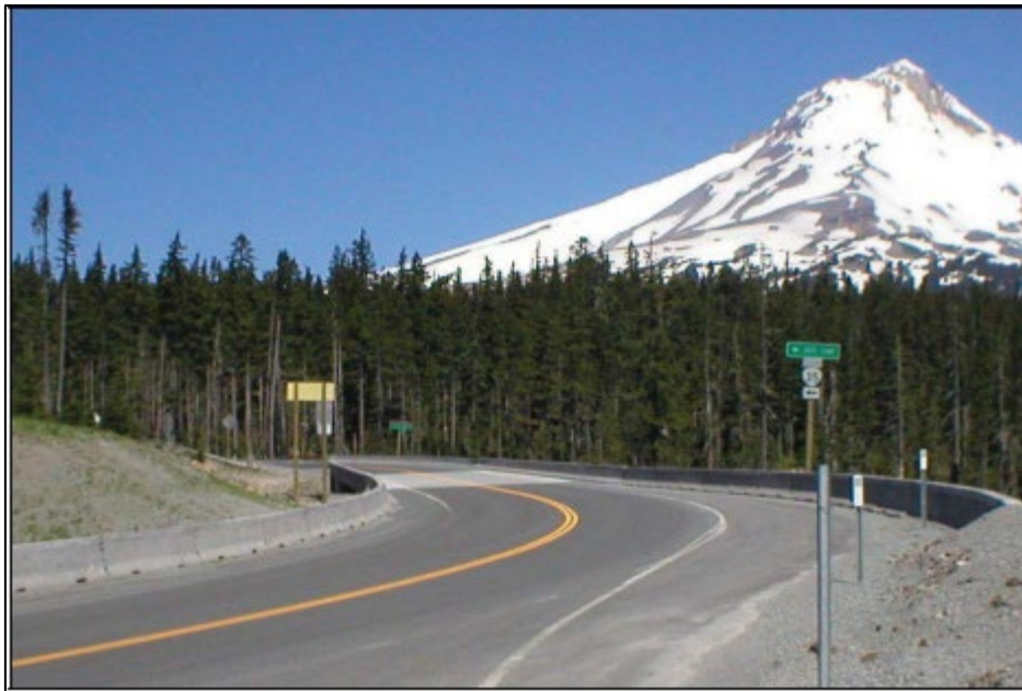
Figure 96. Photograph. Example concrete safety shape. (59)
