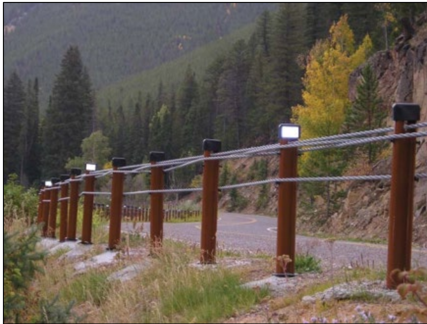
Figure 73. Photograph. Example high-tension cable. (59)
