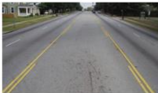
5 lane roadway with wide lanes, no bike lanes
