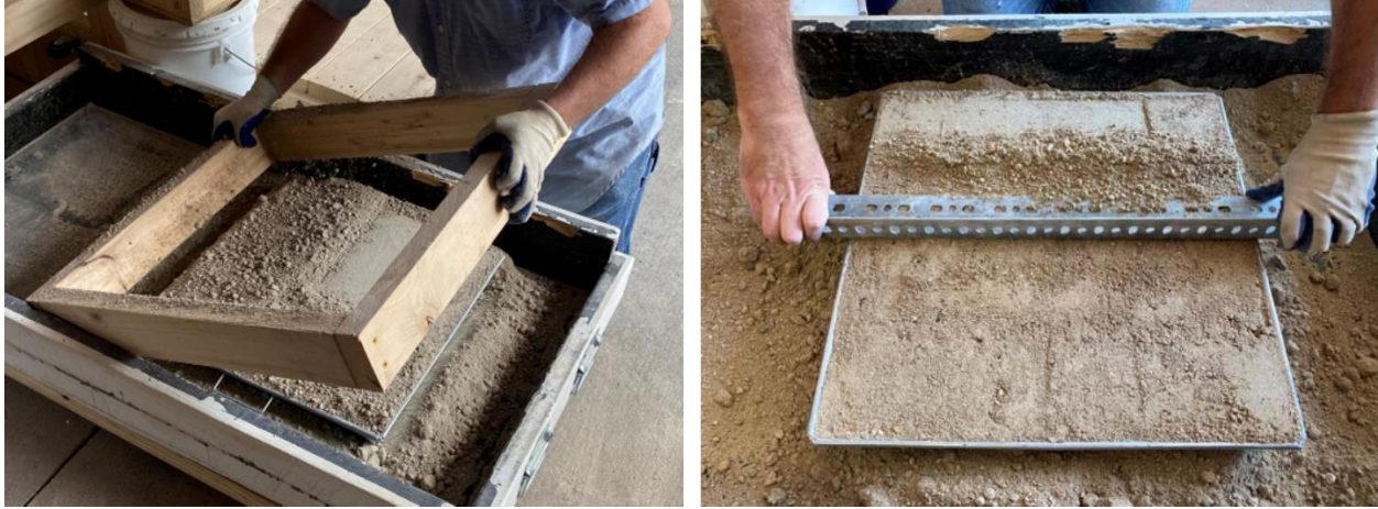
Figure 37. Preparation and screeding of compacted soil form
