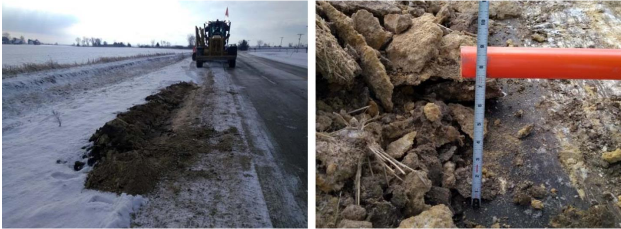
Figure 27. Motor grader and soil sampling from CR Z24 in Clinton County
