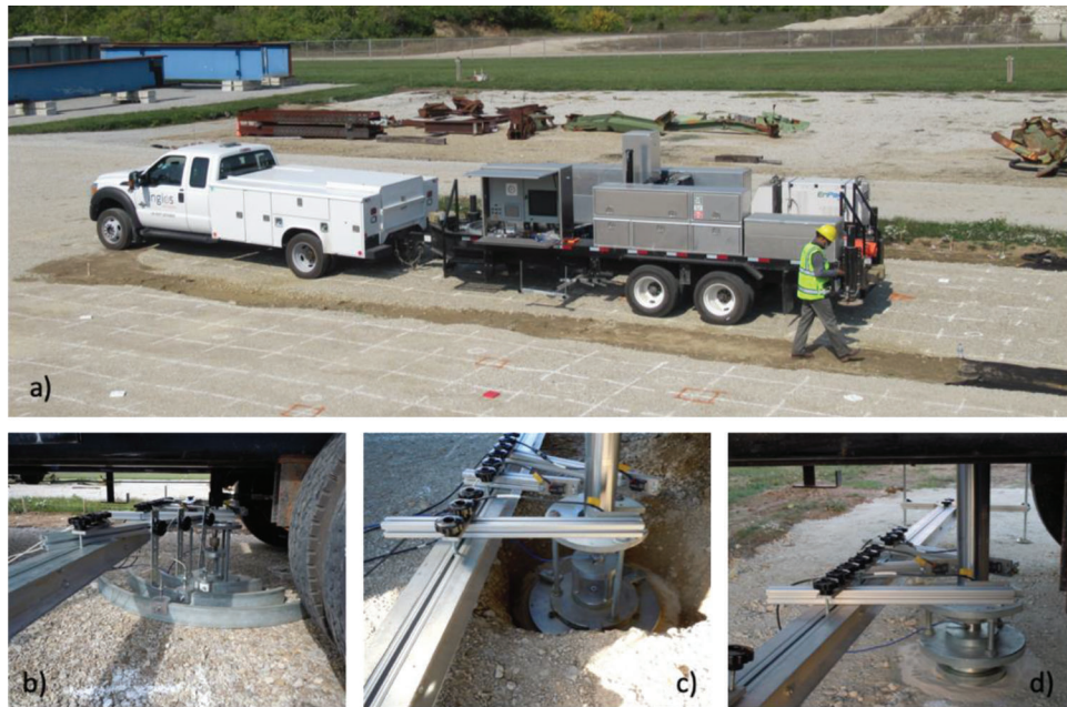
Figure 3.14 (a) APLT trailer and setup for automated plate load test (APLT), (b) on aggregate subbase with multi-radii deflection measurements, and (c) on subgrade after removal of aggregate, and (d) setup for static load tests.
