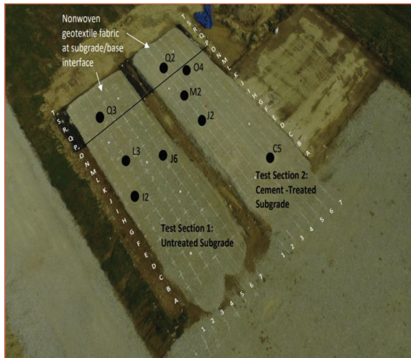
Figure 3.3 Plate load testing locations on S-BRITE strips.
