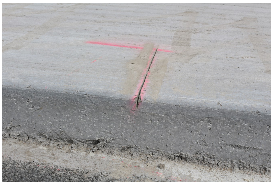
Figure 3. Photo. Active crack control saw cut notch.
