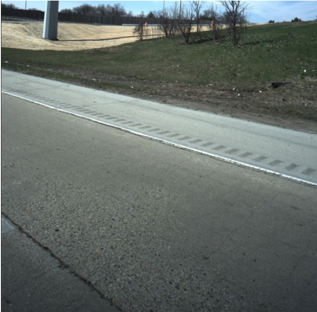
Figure 10. Image. IROADS image of transverse cracks in right driving lane with light pole, pavement stripes, shoulder grooves, and pavement width as reference distances.
