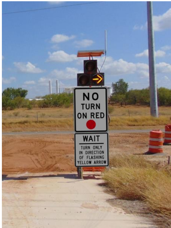
Figure 22. Proceed Right Three-Section Doghouse DAD.
