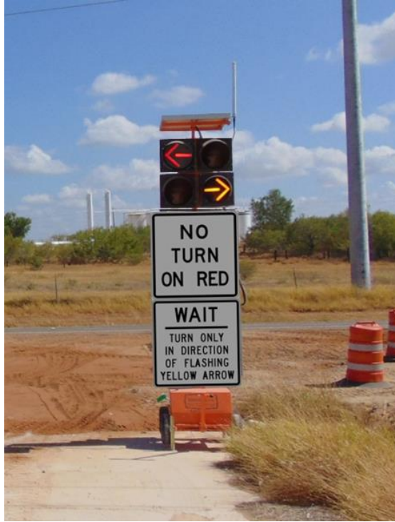
Figure 25. Proceed Right Four-Section Stacked DAD.
