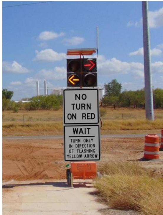
Figure 24. Proceed Left Four-Section Stacked DAD.
