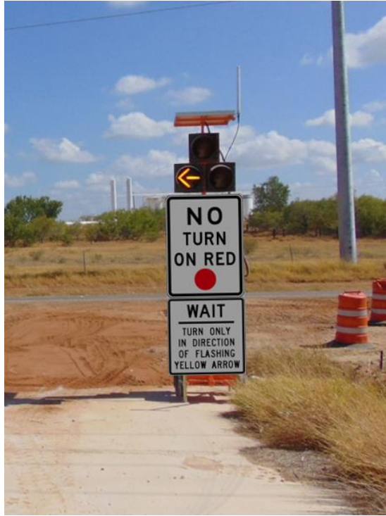
Figure 21. Proceed Left Three-Section Doghouse DAD.
