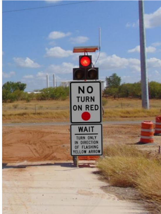
Figure 23. Stop Three-Section Doghouse DAD.
