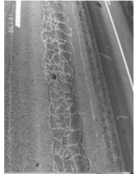
Figure 2. Example of Pavement Roughness in Fatigued Test Sections
