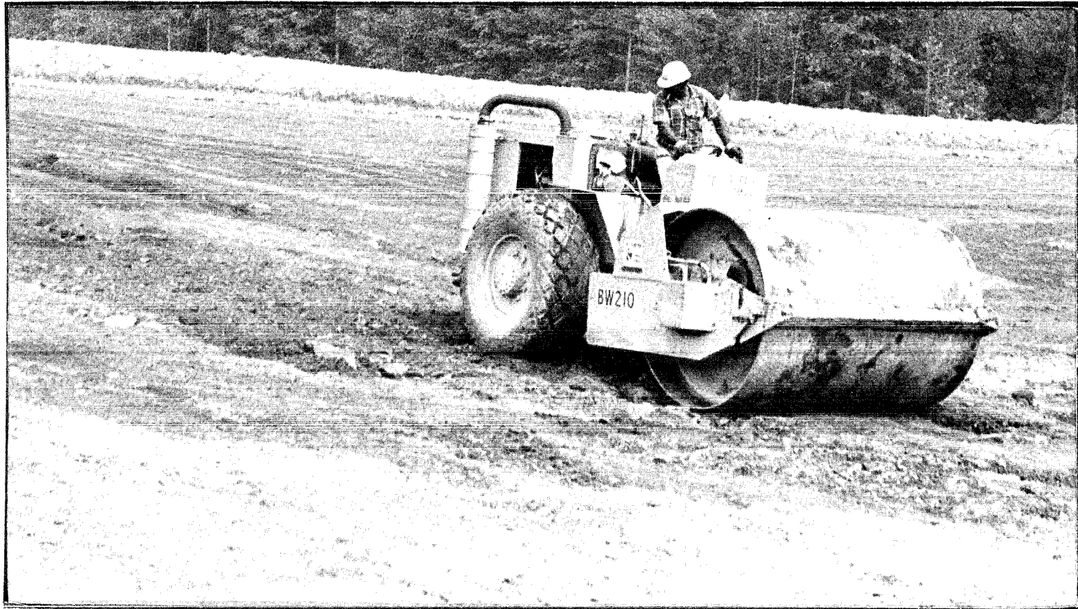
Figure 11. Compacting of Coarse Coal Refuse using a Barmac Vibratory Compactor, BW 210 with Earthen Containment Structure in Background.
