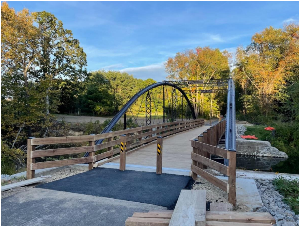
Figure 2: A rehabilitated Messerall Road Bridge at its new location over Linesville Creek, on the Pymatuning State Park Spillway Trail. (Source: PennDOT)
