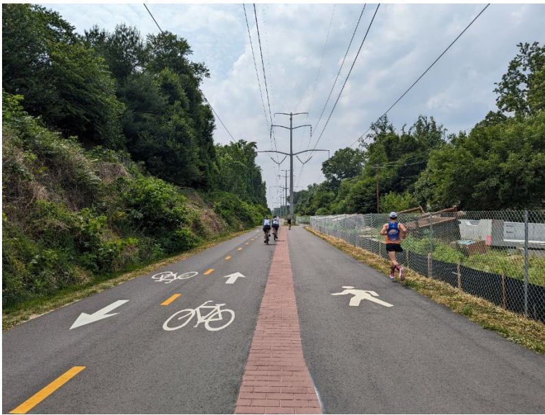
Figure 2: On behalf of the Northern Virginia Regional Park Authority, NVTA funded a project through the city of Falls Church to create a “dual” on a busy segment of the Washington and Old Dominion regional trail, providing separate lanes for pedestrians and bicyclists. Source: NVTA
