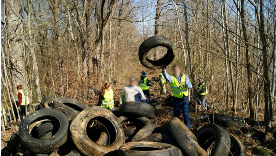
Figure 6: Volunteers removing dumped tires to use for the Tires to Trails project. Source: TN Department of Environment and Conservation, TTSP
