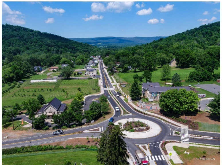
Figure 1: In rural Loudoun County, NVTA funded the Route 9 traffic calming project through the town of Hillsboro, featuring enhanced sidewalks, crosswalks, and roundabouts. Source: Town of Hillsboro, Virginia
