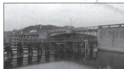
A bridge over the St. John's River in Florida.
