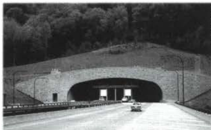
FHWA's new Tunnel Management System will help agencies manage tunnels such as the one shown above.
