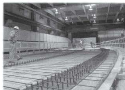
Reinforcing steel is placed before the concrete deck is poured.
