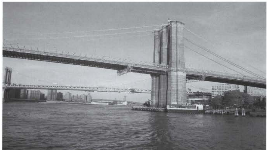
FHWA's new Bridge Program Technology Deployment Teams will create action plans for delivering technology and technical assistance to State highway agencies responsible for developing and managing bridges.
