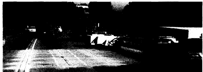
The Balsi Beam, deployed here in a work zone, provides an enclosed safety zone for construction.
