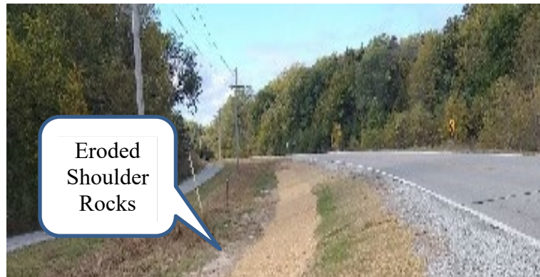
Figure 1.1 Crushed Rock Surface at Hwy 31 (Rocks in the shoulder were washed out.)
