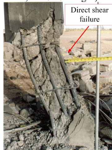
(c) Blast test [38]
