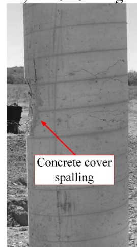
(c) Blast test [29]
