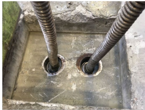
(c) Second concrete base
