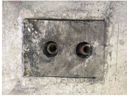
(a) First concrete base
