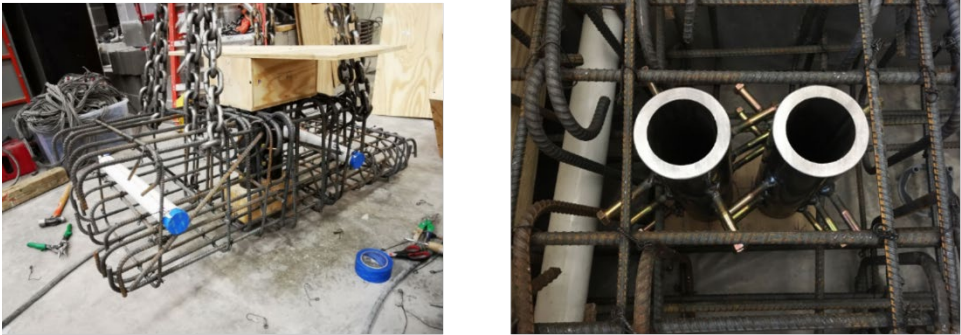
Figure 3.18 Inside of the second concrete base
