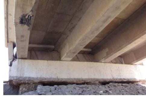
(b) Chada bridge with no diaphragms, Chile
