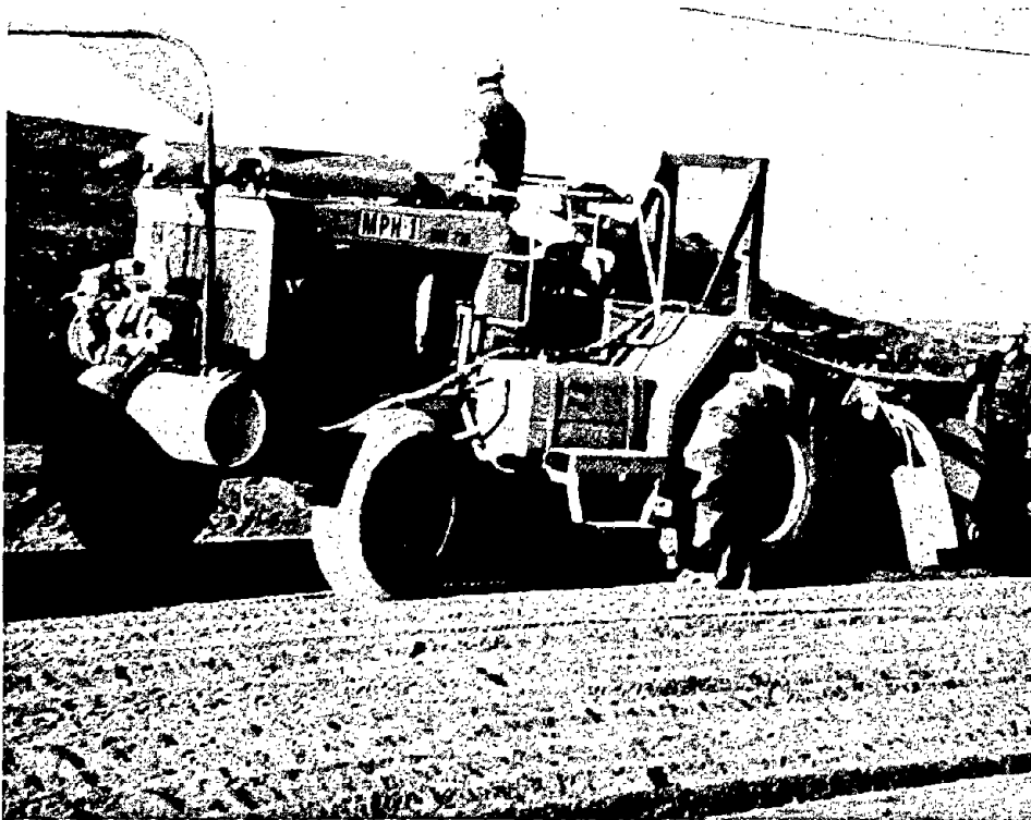
Figure 23. Multiple transverse shaft rotary mixer (flat type) (51).
