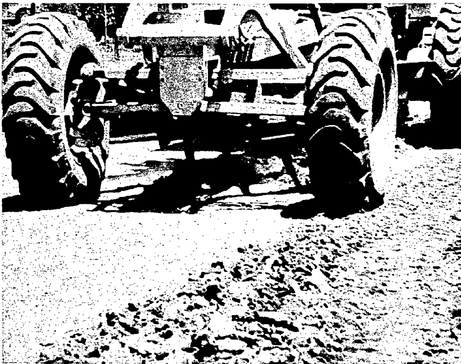
Figure 27, Scarification with motor grader (47).
