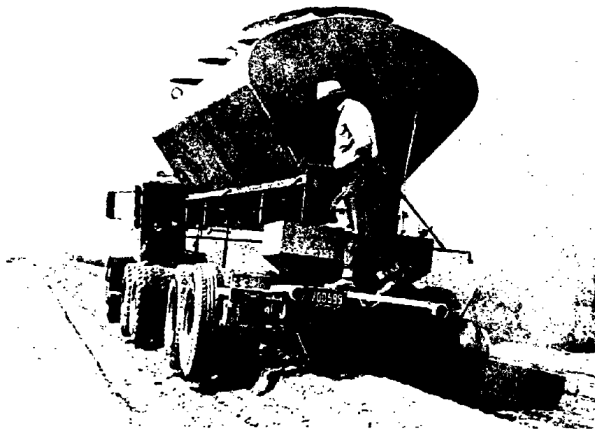
Figure 42. Windrow-type mechanical spreader is used to place cement on top of windrow of soil (51).
