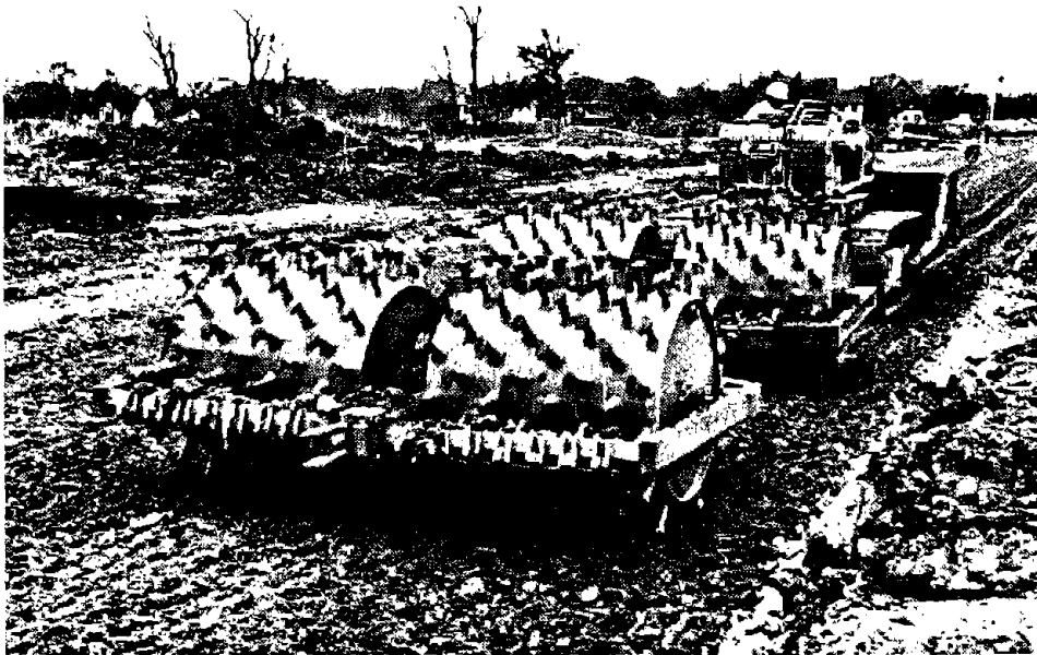
Figure 35. Initial compaction of lime-soil mixture with sheep's foot roller (47).
