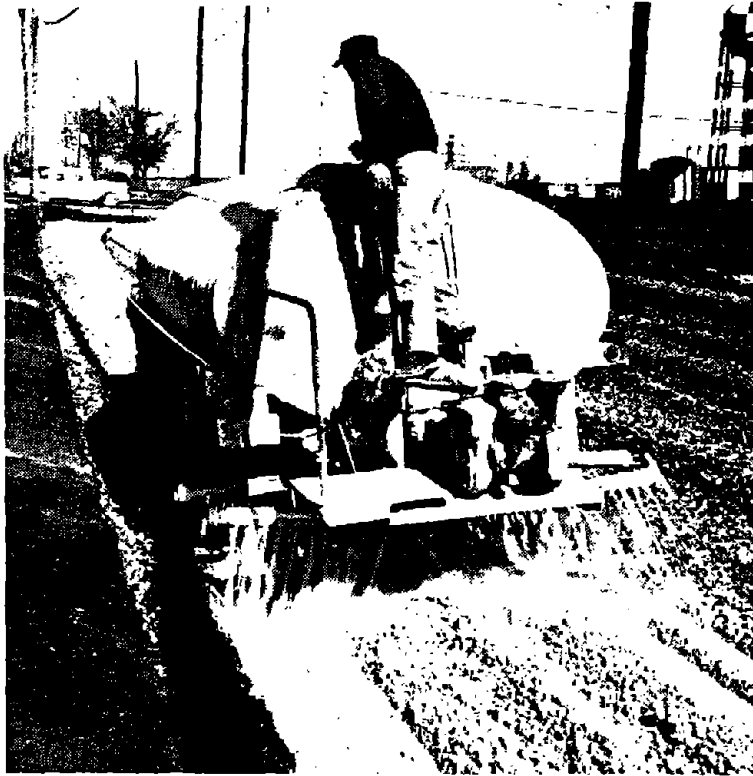
Figure 31. Transit mixing of lime slurry on city street project, using recirculating pump at rear. Pressure and gravity spray bars distribute lime evenly (47).
