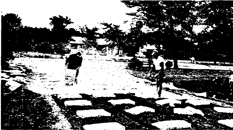
Figure 28. Bagged lime application showing bag spacing for 4% distribution on worn-out city street (47).
