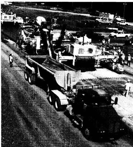
A two-lift concrete pavement test section under construction in Pleasanton, KS, in June 2008 on U.S. 69 and East 1100 Road.
