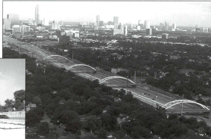
Left and above: The Houston Gateway project replaced four bridges spanning the US 59-Southwest freeway.
