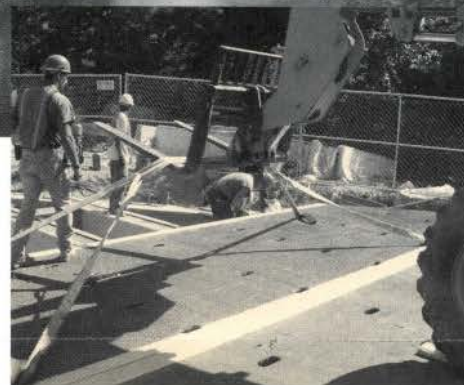
Inset right: The Maryland State Highway Administration replaces the deck on a steel through-truss bridge on MD Route 24 with an FRP composite deck. The photo above shows the completed bridge.
