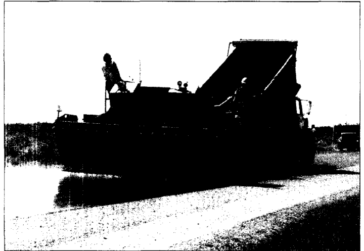
One of the preventive maintenance treatments being championed by the new Midwestern Pavement Preservation Partnership is chip sealing, which is shown here.
