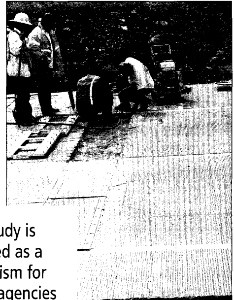
A weigh-in-motion system is installed on I-40 near Flagstaff, Arizona.
