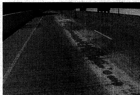
Left: Diamond grinding is performed on the longitudinal construction joint in the left wheel path of a bridge deck on U.S. 23 in southern Ohio. Right: The bridge deck after diamond grinding was performed, greatly improving ride quality.
