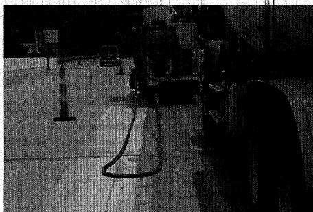
Left: Diamond grinding is performed on the longitudinal construction joint in the left wheel path of a bridge deck on U.S. 23 in southern Ohio. Right: The bridge deck after diamond grinding was performed, greatly improving ride quality.
