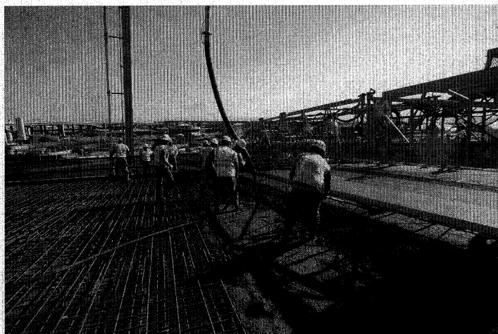
Concrete is poured for the new I-580 connector ramp.
