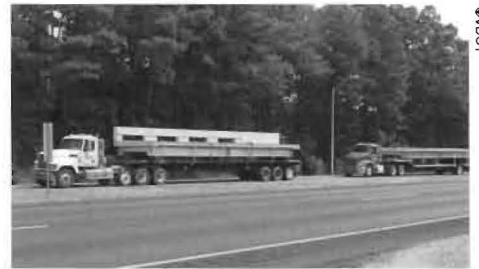
Projects that have used accelerated bridge construction include the Virginia Department of Transportation's replacement of the superstructure of a bridge on Route 15/29 in Prince William County. At top is the completed bridge. The bridge's superstructure segments were fabricated off site (bottom).
