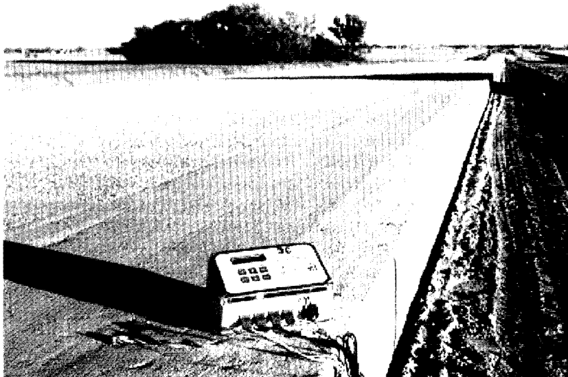
This Maturity Meter is measuring the pavement's compressive and flexural strength.
