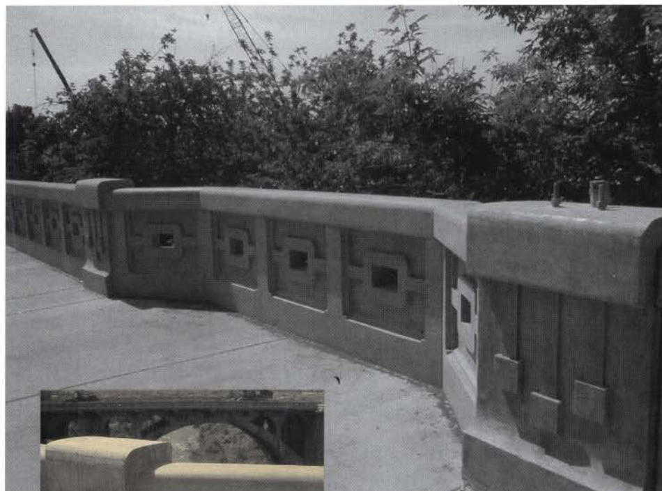
The photos above and at left show an SCC bridge railing constructed in Spokane, Washington. Below is an SCC box segment.
