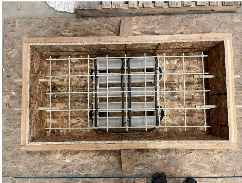
Figure 3.6 Plan View of GFRP Rebar Test Slab
