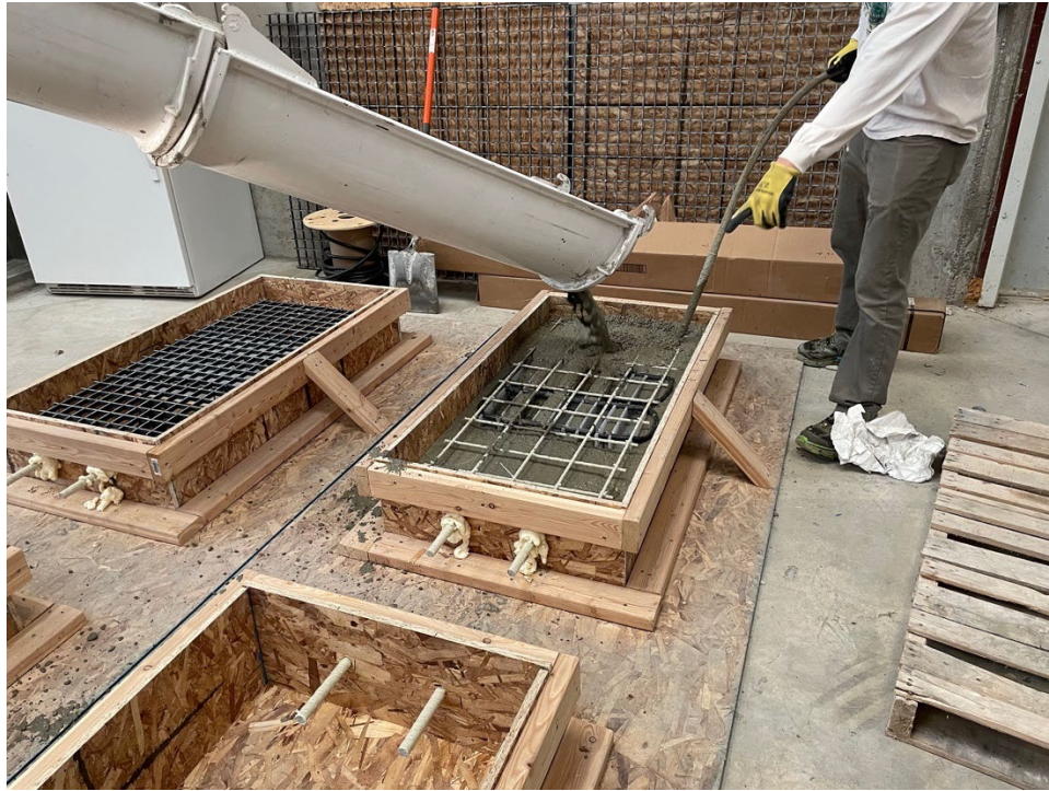
Figure B.2 Filling the GFRP Rebar Form with Concrete
