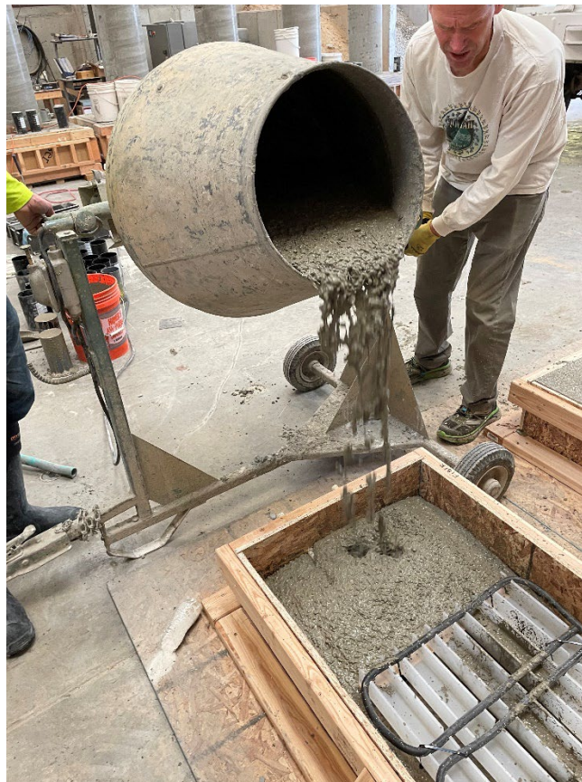
Figure 3.10 Pouring FRC Test Slab from Drum Mixer
