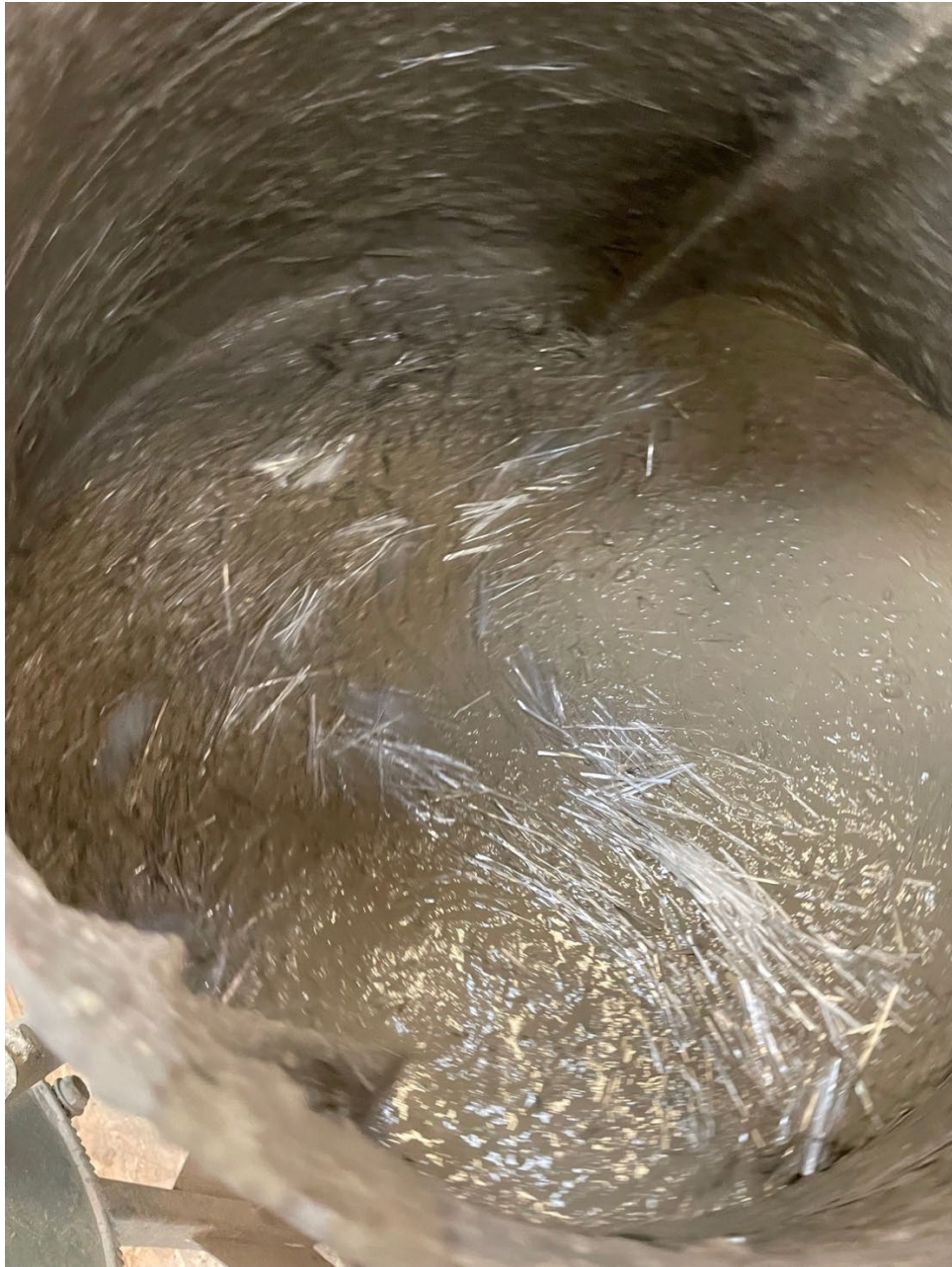
Figure B.3 Adding Macro Fibers to Concrete Drum Mixer
