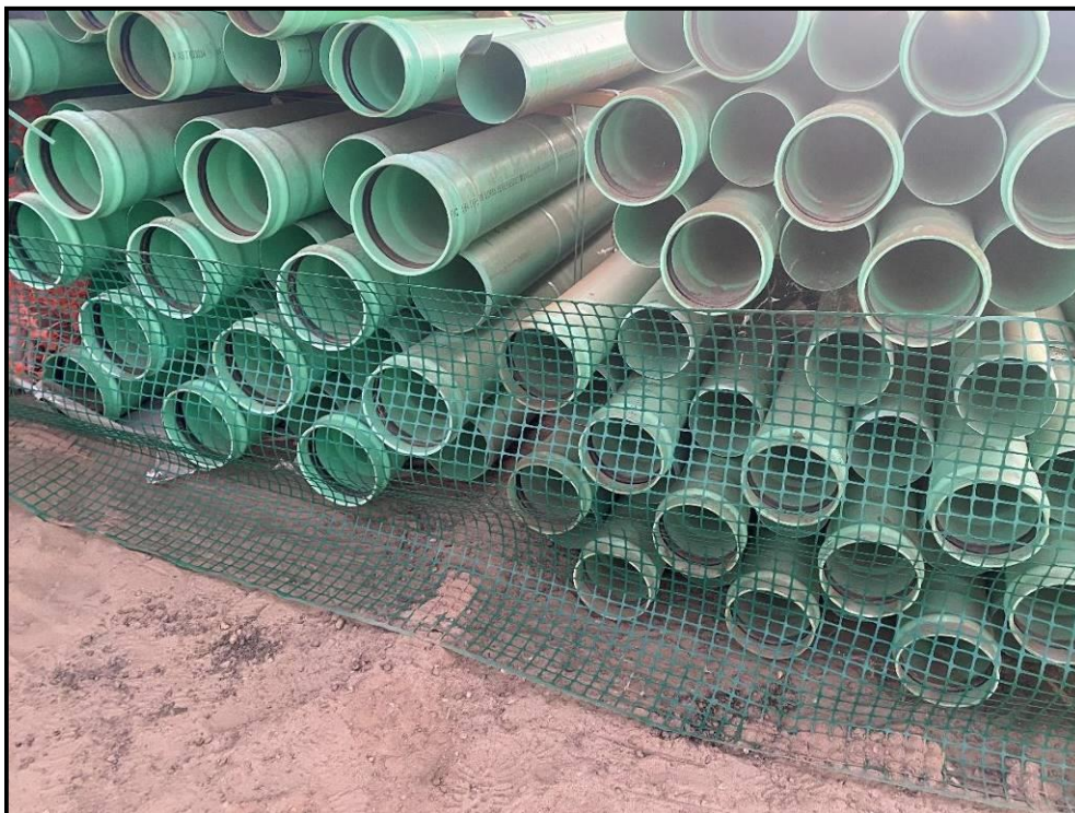
Figure 23. Plastic fencing around construction materials on the Mercy Southwest Hospital study site, Bakersfield, CA, January 2024. (Photo by E. Noel)
