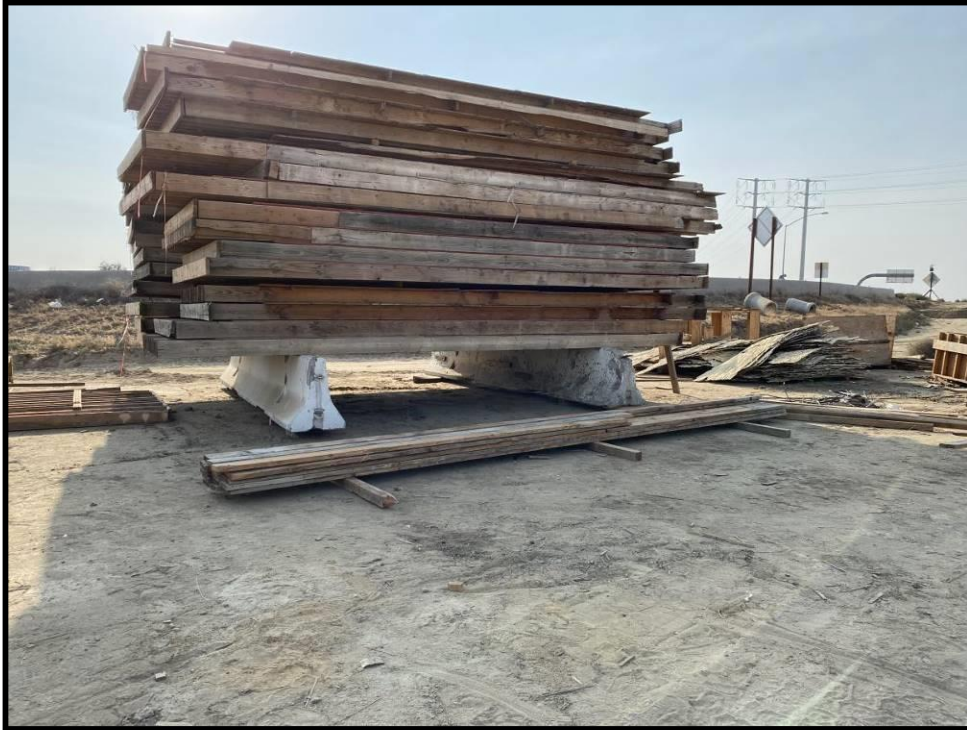
Figure 6. Construction materials placed up on K-rails on the Centennial Corridor road construction site in Bakersfield, CA. (Photo by E. Noel)
