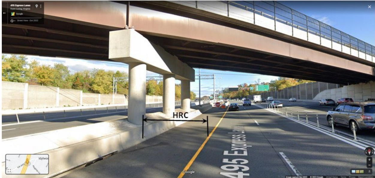
Figure 2-1. Photo. Example of a horizontal roadside clearance.
