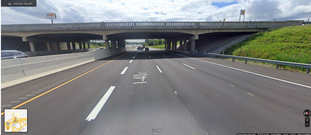
Original Photo: © 2022 Google® (see Acknowledgments page) Figure 2-36. Photo. Street view of Mt. Juliet Road bridge over I-40.
