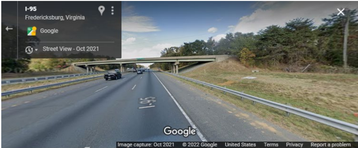
Figure 3-24. Photo. Example of Low curvature of driving lane below structure.
