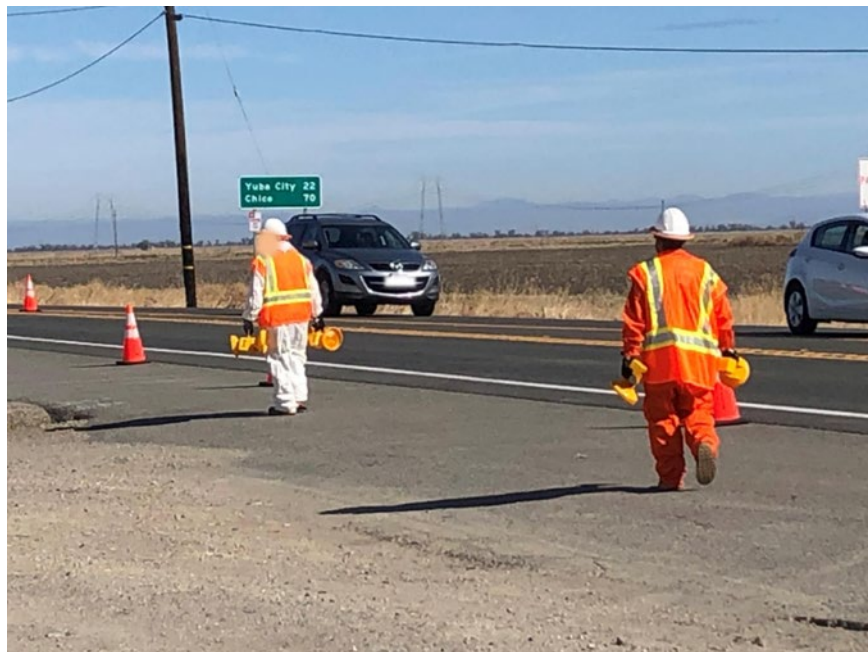
Figure 5.25 Retrieval of Intellicone System at the end of Trial
