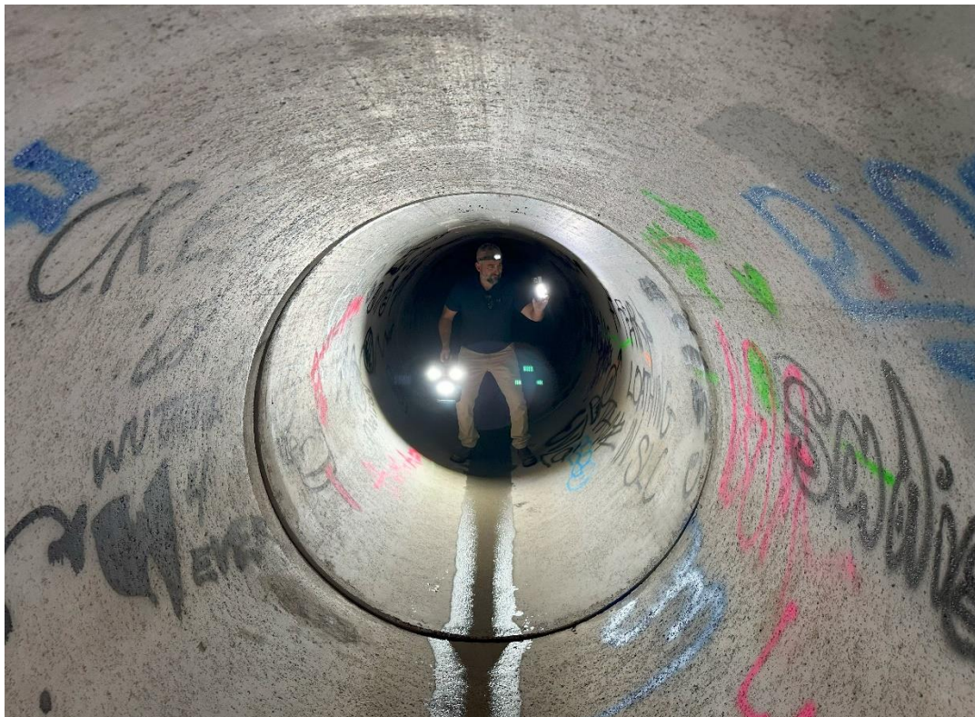
Figure 3.3.1 Herriman Tunnel – John Caya, Scanning with Pocket LiDAR
