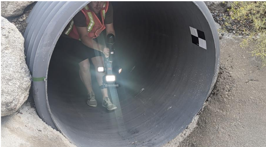
Figure 3.4.1 - Brady Reisch using Leica BLK2GO Mobile Lidar Scanner Lisa Falls Cross Culvert, Little Cottonwood Canyon, August 21, 2023
