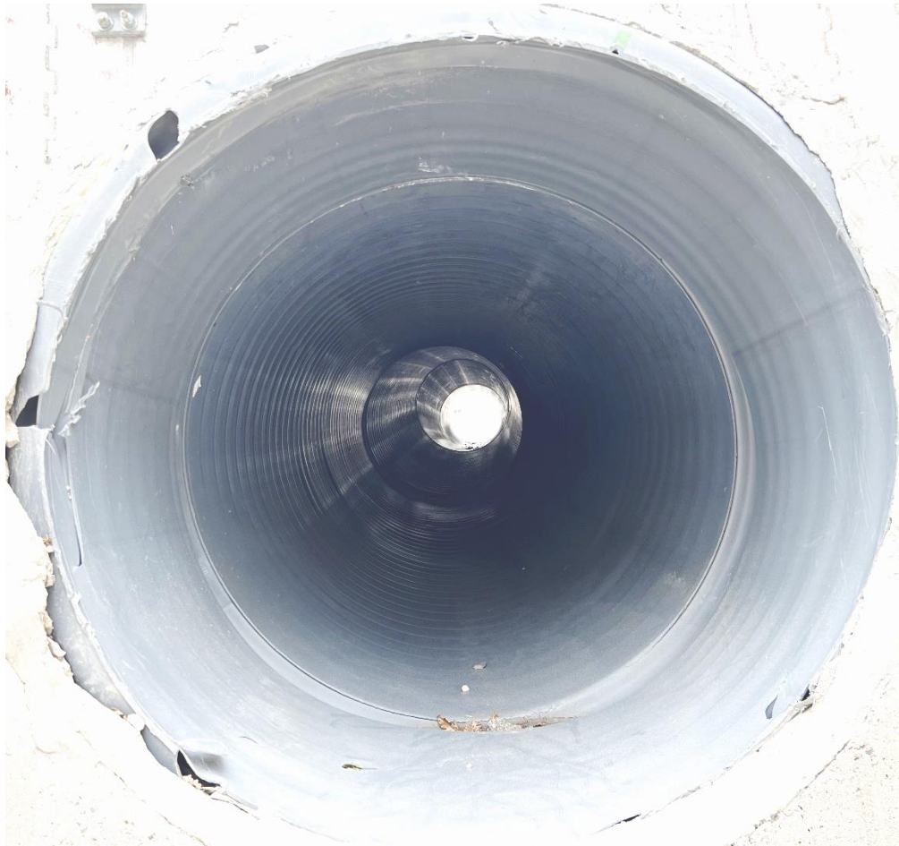
Figure 4.7.1 – Photo of Interior Grade Change, Lisa Falls 60” Polypropylene Pipe
