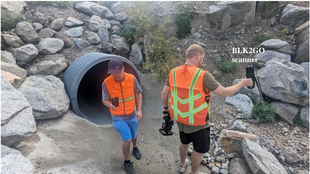
Figure 2.6.1 Photo of Brady Reisch using Leica BLK2GO Mobile LiDAR Scanner to create 3D scan of Lisa Falls Cross Culvert, Little Cottonwood Canyon, August 21, 2023
