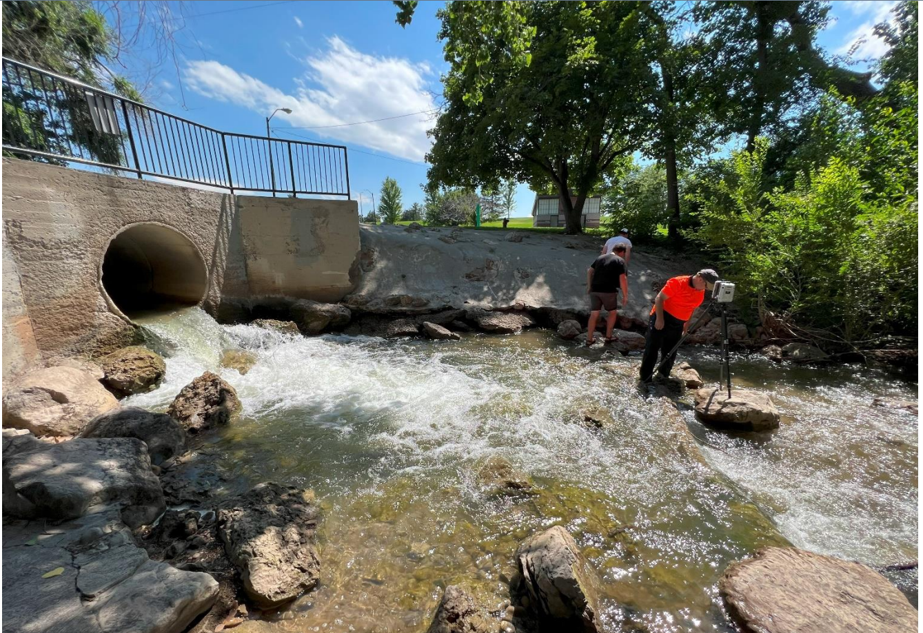
Figure 3.12.1 – Sugarhouse Park, Reinforced Concrete Pipe, Michael Olsen, Aaron Mackliet and Daxton Nielson scan the outlet/headwall with the RTC360 Scanner, August 8, 2023
