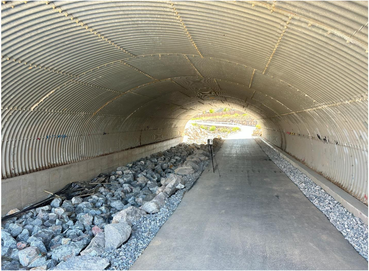
Figure 3.2.1 Herriman Midas Creek – Culvert with RTC360 Scanner Shown
