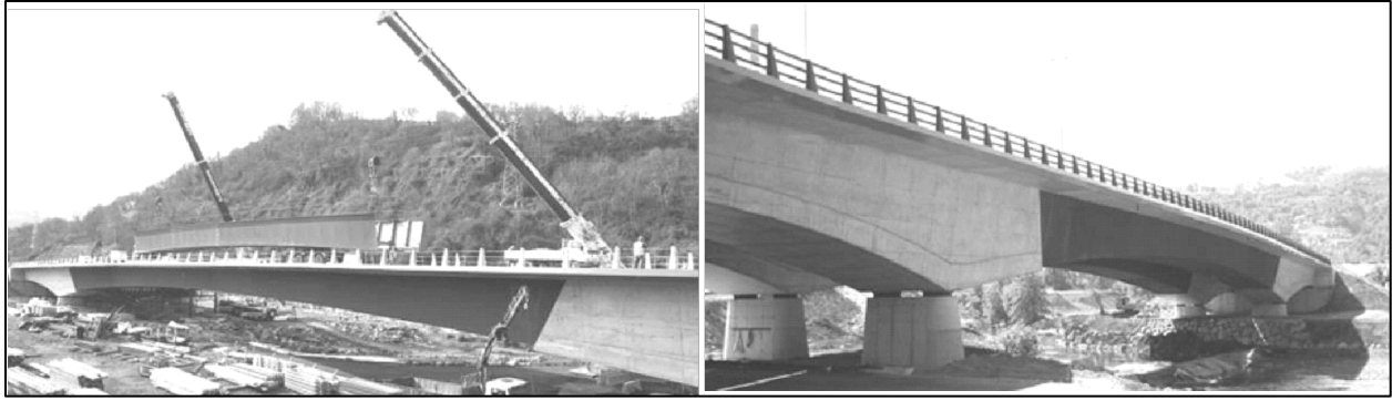
Figure 2.15 Nalón River in Langreo bridge, Spain (PAÑTAK 2012)
