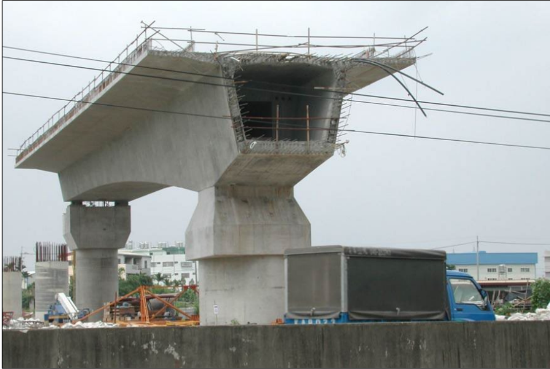
Figure 2.3 Example of concrete box girder bridge (Wordpress 2015)
