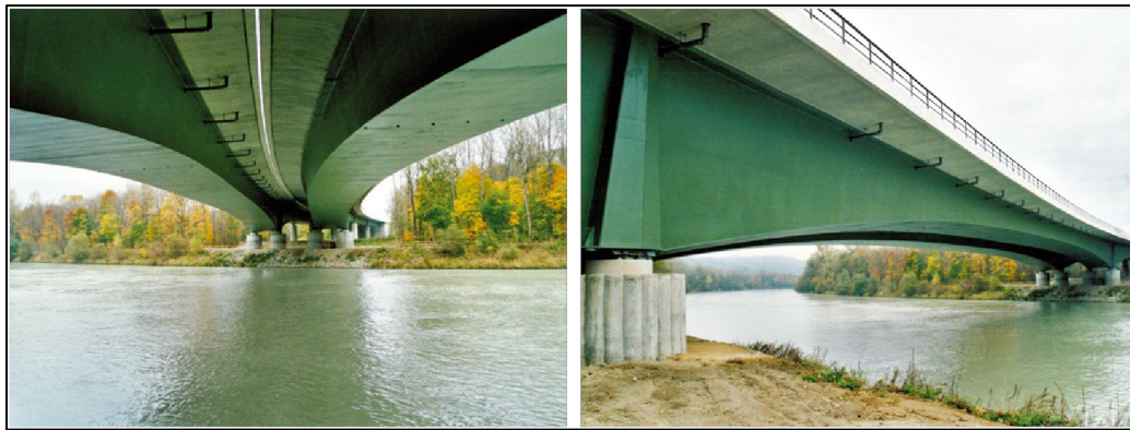
Figure 2.14 Inn River in Neuötting bridge, Germany (PAÑTAK 2012)
