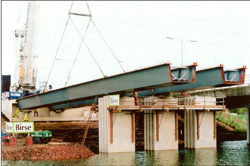
Figure 2.4 Example of steel box girder bridge (SteelConstruction.info 2019)
