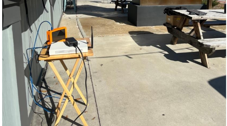
Figure 29. Photo. The field test setup from a different angle
