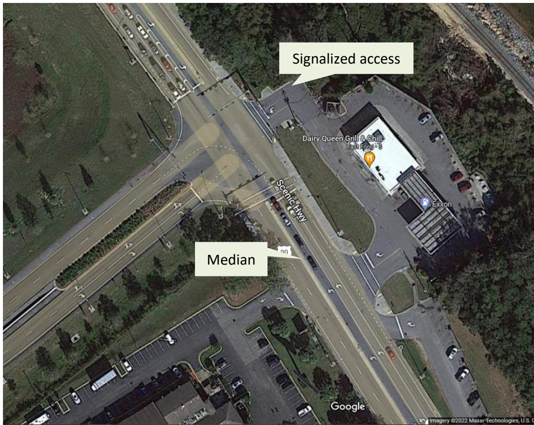
Figure 72. Driveway access as reconstructed in 2016.
