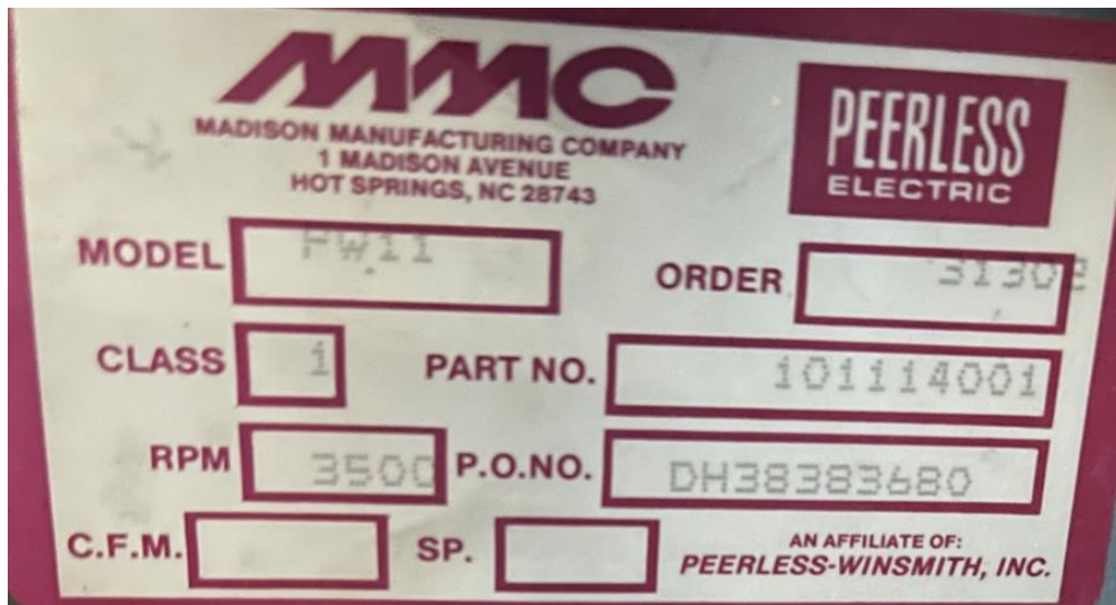
Figure 7. Inlet air sample blower nameplate
