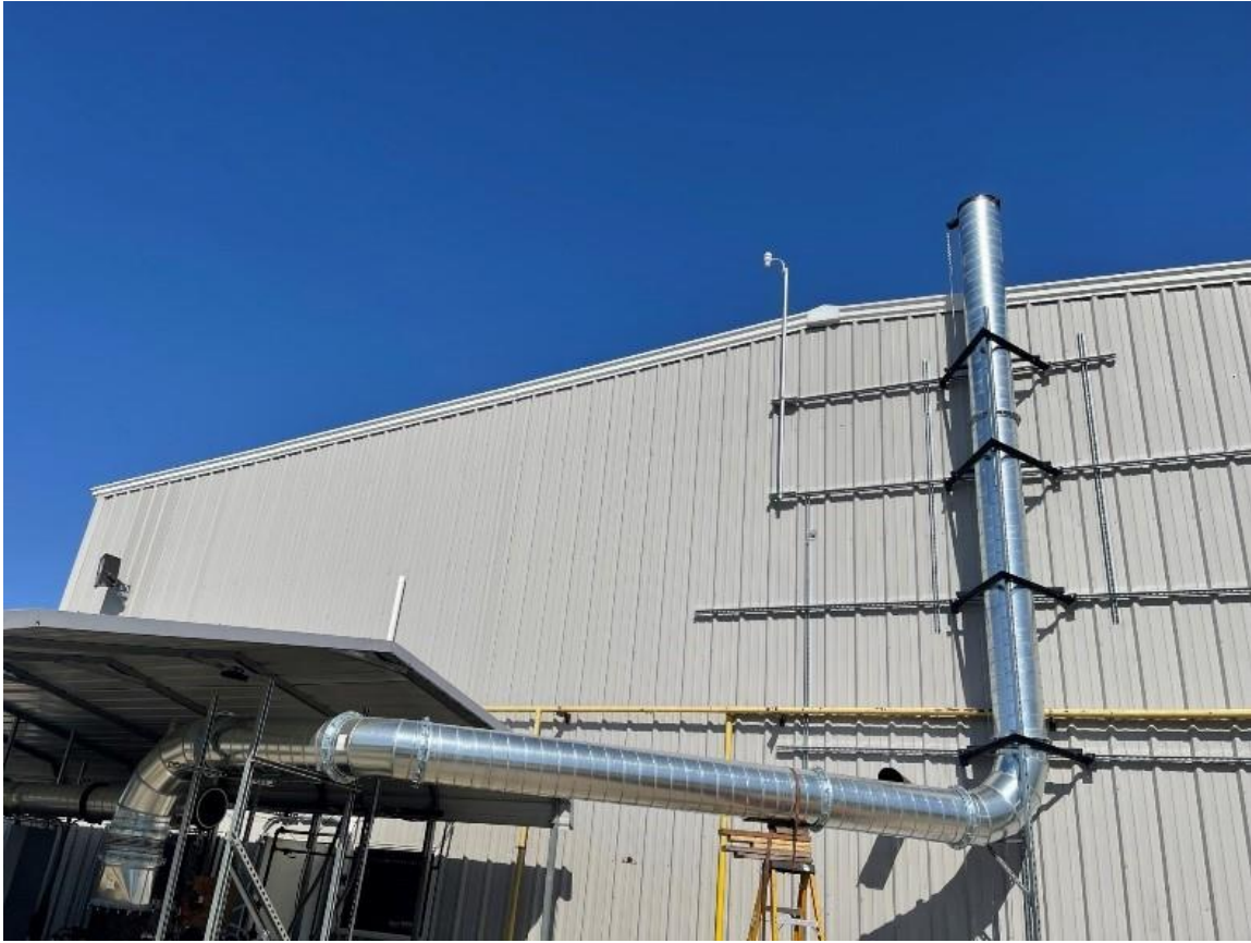
Figure 8. Engine exhaust system
