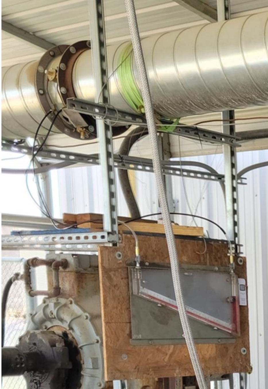
Figure 6. Dwyer Series 424 stationary gage flowmeter
