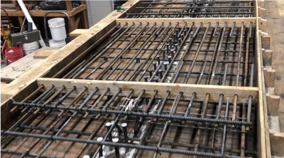
Figure 15. Reinforcement in the link slab
