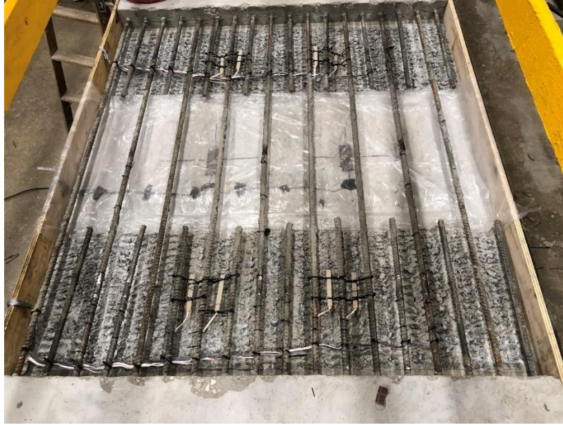
Figure 16. Instrumentation and debonding of the link slab portion
