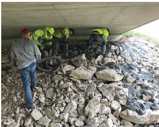
Grout placement under an existing bridge in Buchanan County
