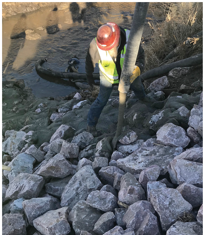
Grout placement prior to bridge construction at a Woodbury County site
