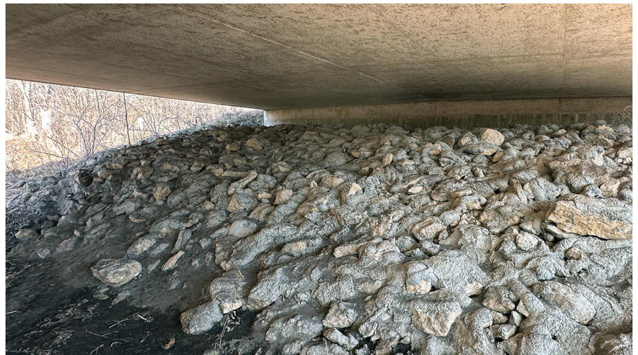
Partially grouted revetment under a low-volume bridge
