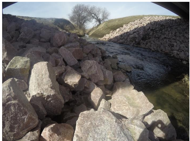
Figure 23. Recently installed loose riprap in good condition in Woodbury County, Iowa
