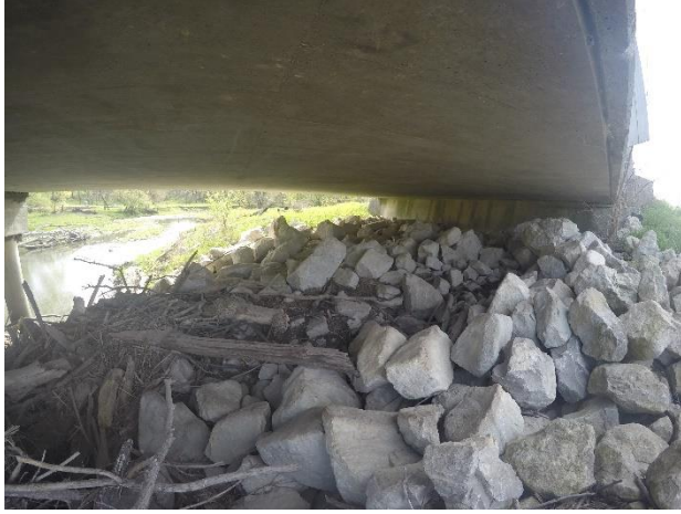
Figure 30. Loose riprap and failing fabric in poor condition in Madison County, Iowa
