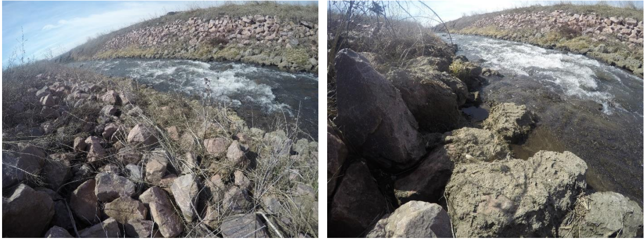
Figure 24. Partially grouted riprap in Woodbury County, Iowa
