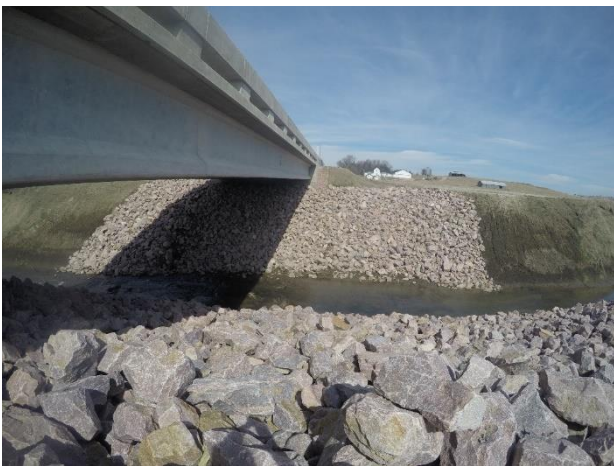
Figure 23. Recently installed loose riprap in good condition in Woodbury County, Iowa
