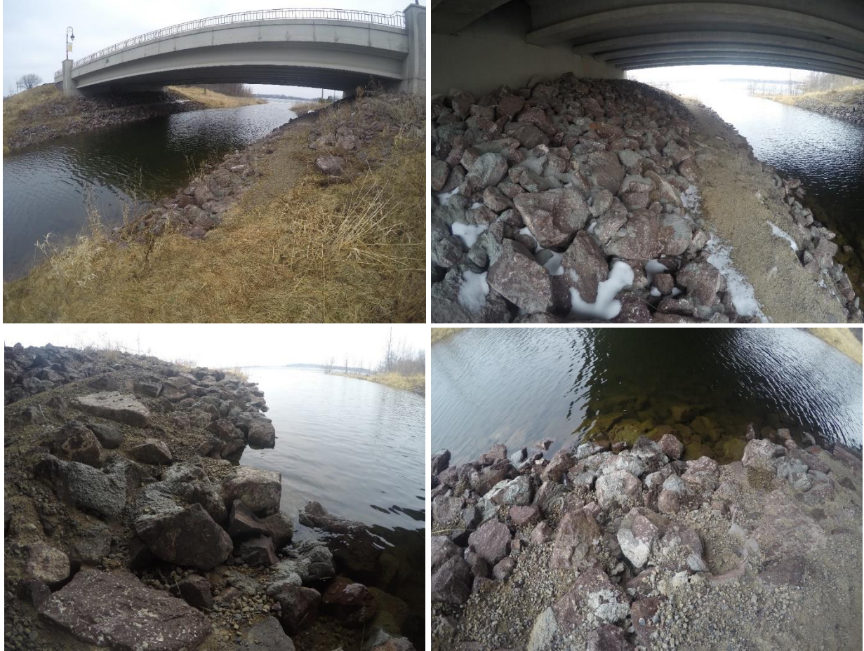
Figure 17. Minnesota Site 2: Partially grouted riprap
