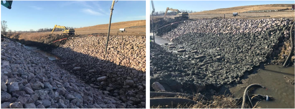
Figure 43. Woodbury County site before (left) and after grouting (right)
