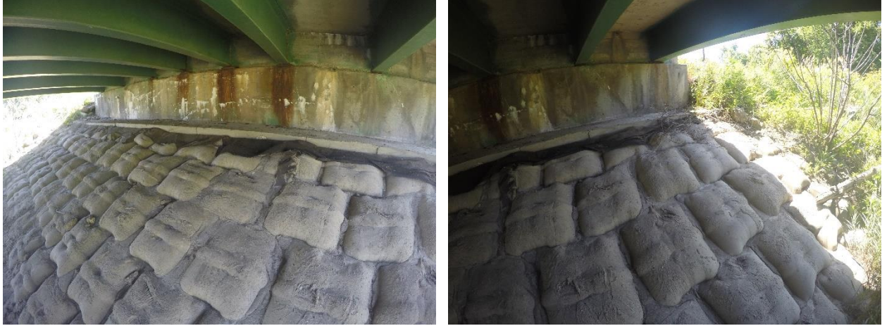
Figure 27. Grout-filled blankets in Buchanan County, Iowa
