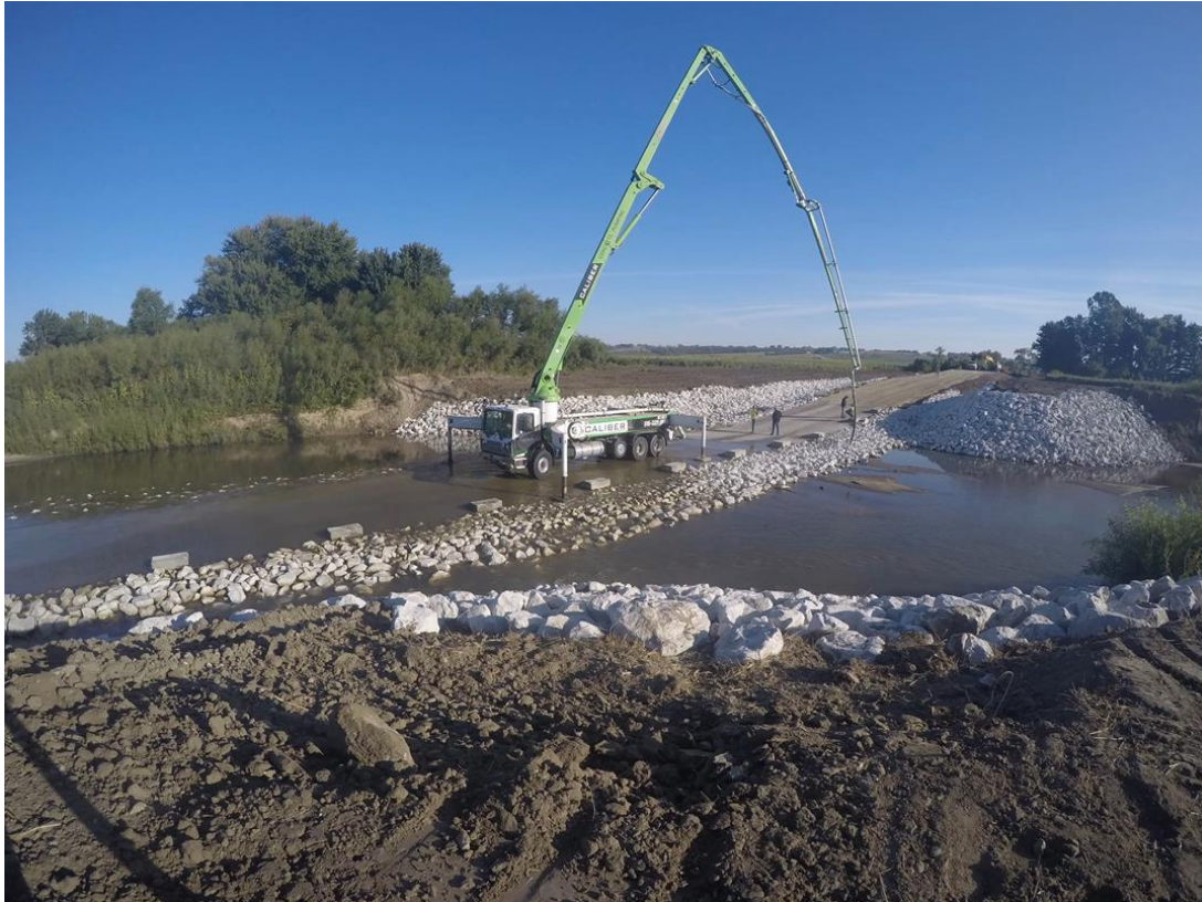
Figure 37. Low water crossing installation site in Madison County with pump shown
