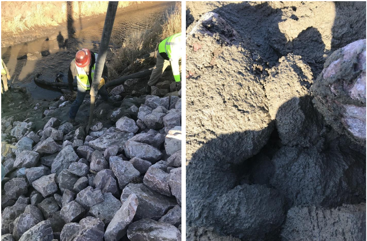
Figure 44. Woodbury County grouting (left) and grout consistency (right)
