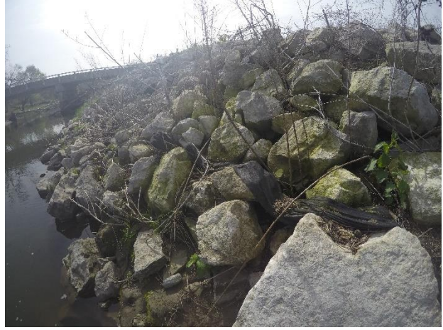
Figure 30. Loose riprap and failing fabric in poor condition in Madison County, Iowa
