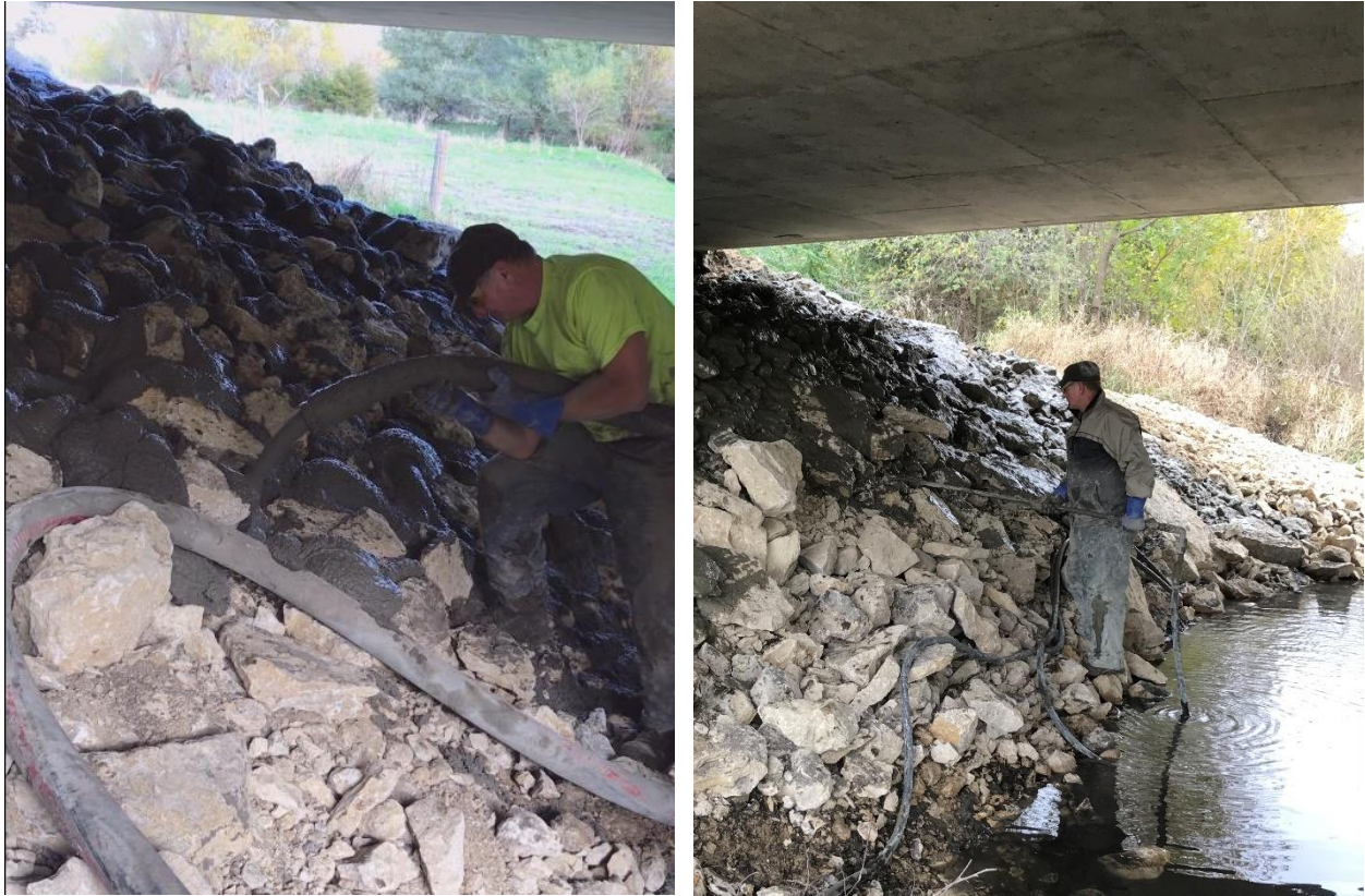
Figure 35. Grout placement of FHWA mix (left) and Buchanan County grout (right)
