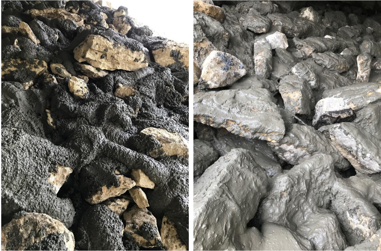
Figure 34. Grout consistency of FHWA mix (left) and Buchanan County grout (right)
