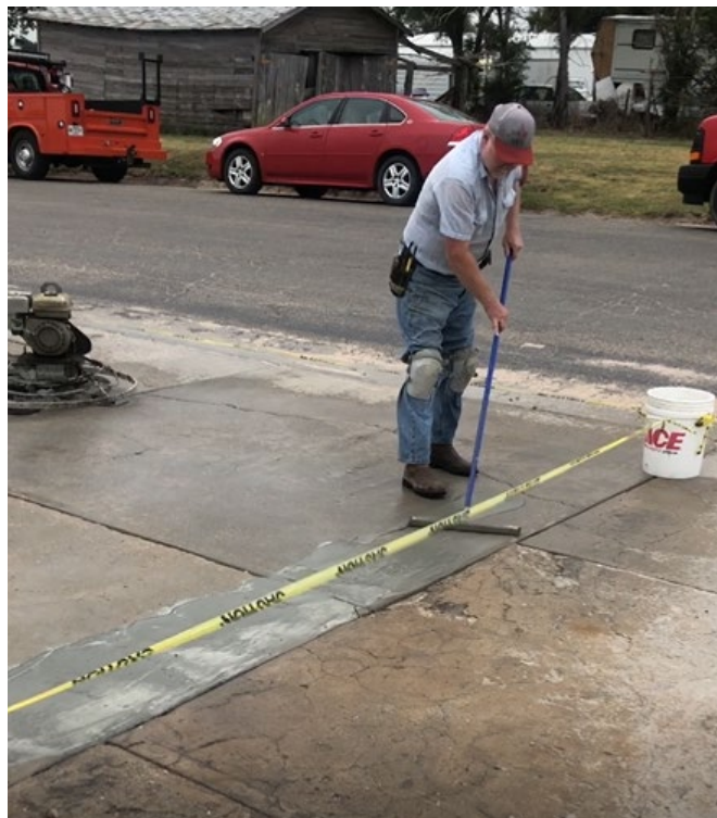
Figure 3.19: Spreading First Layer of JMM with Squeegee
