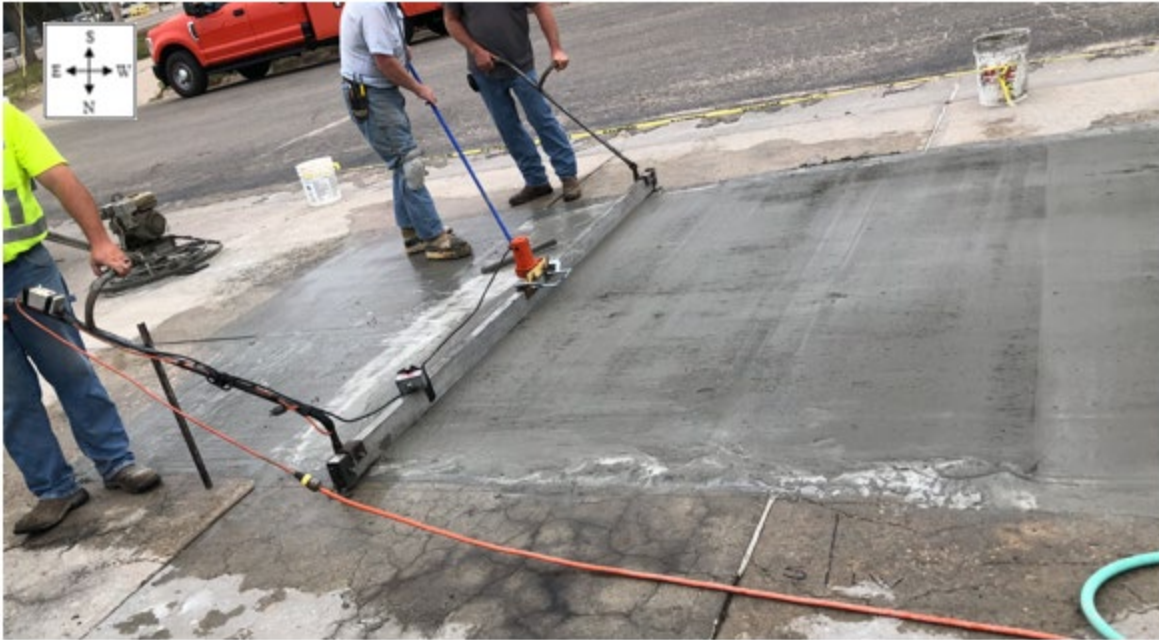
Figure 3.24: Moving Vibrating Screed Along Slab to Consolidate and Smooth JMM
