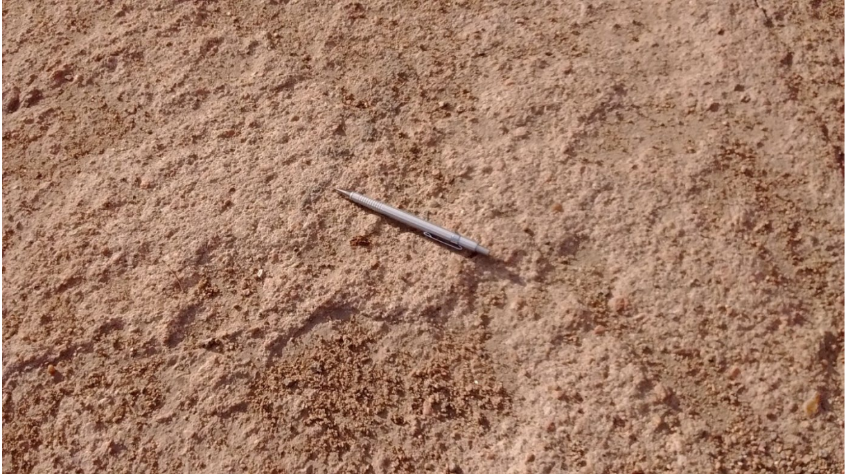
Figure 3.3: Typical Substrate Prior to Overlay Placement
