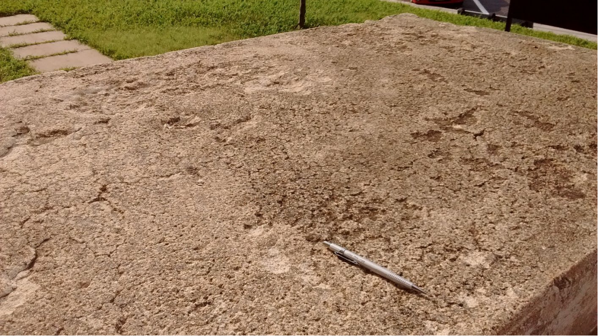
Figure 3.10: Typical Substrate Condition Prior to Topping
