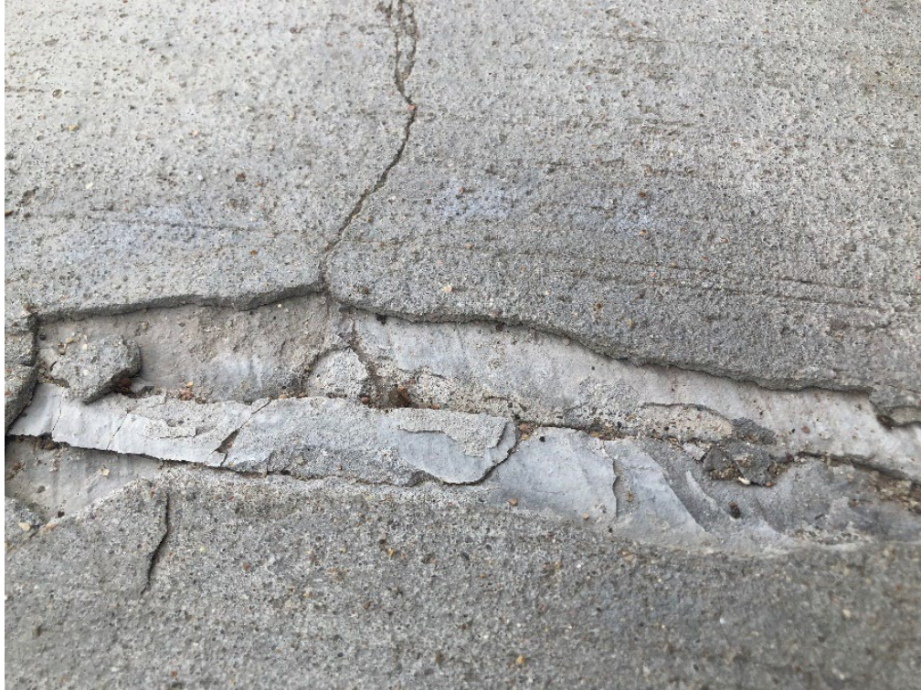
Figure 3.8: Isolated Medium Spall Near Reflected Joint on Sidewalk Showing Underlying Thickness of Each Bonded Layer
