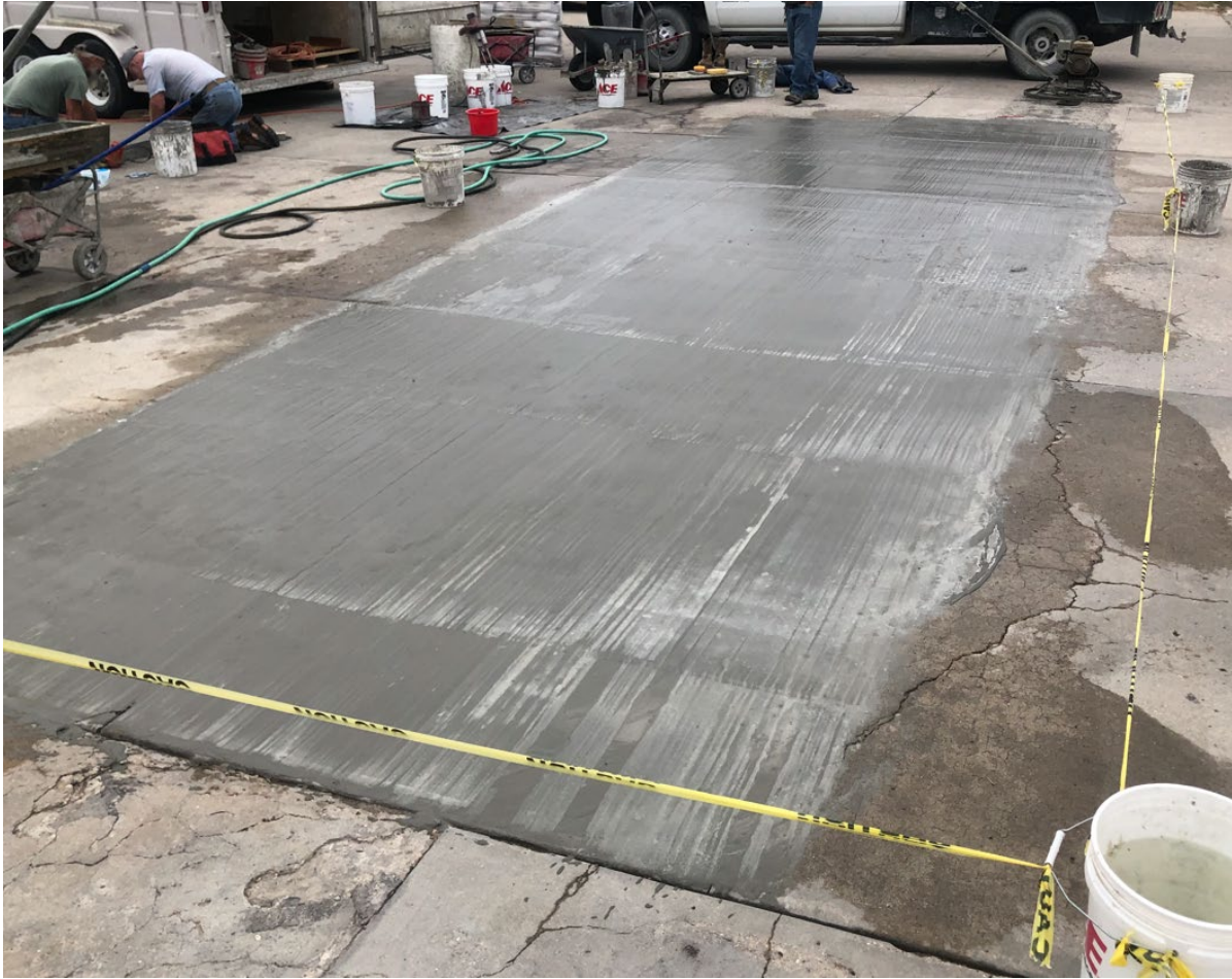
Figure 3.22: Completed First Layer of JMM Overlay
