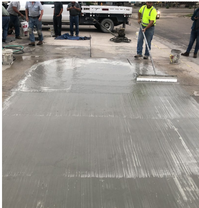
Figure 3.21: Smoothing and Adding Surface Texture with Broom
