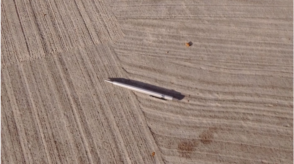
Figure 3.5: Typical Broomed Final Surface Finish of Parking Lot
