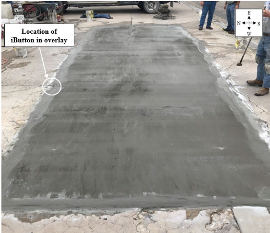
Figure 3.25: Completed Second Layer of JMM Overlay
