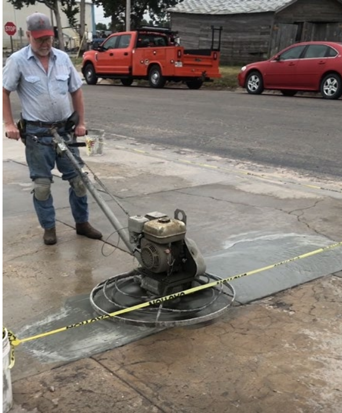
Figure 3.20: Using Power-Trowel to Work JMM into Substrate
