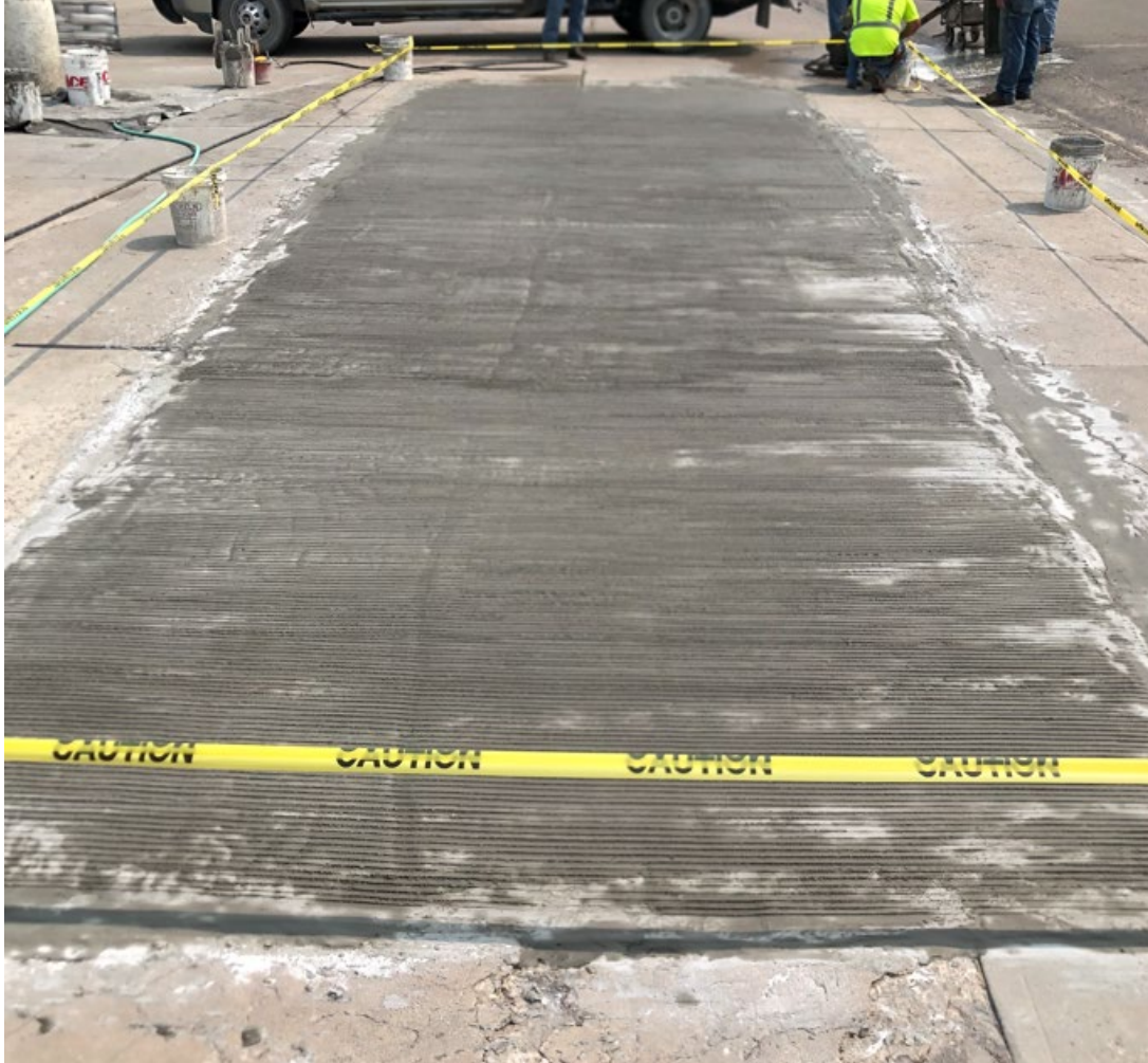
Figure 3.29: Completed Third Layer of the JMM Overlay
