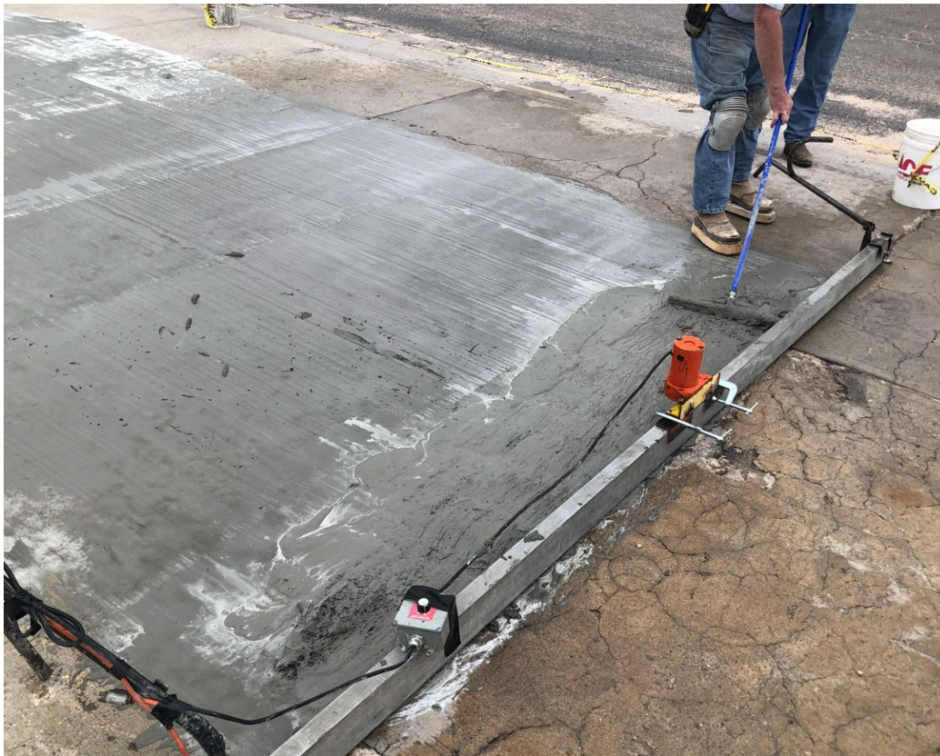
Figure 3.23: Placing JMM in Front of Homemade Vibrating Screed
