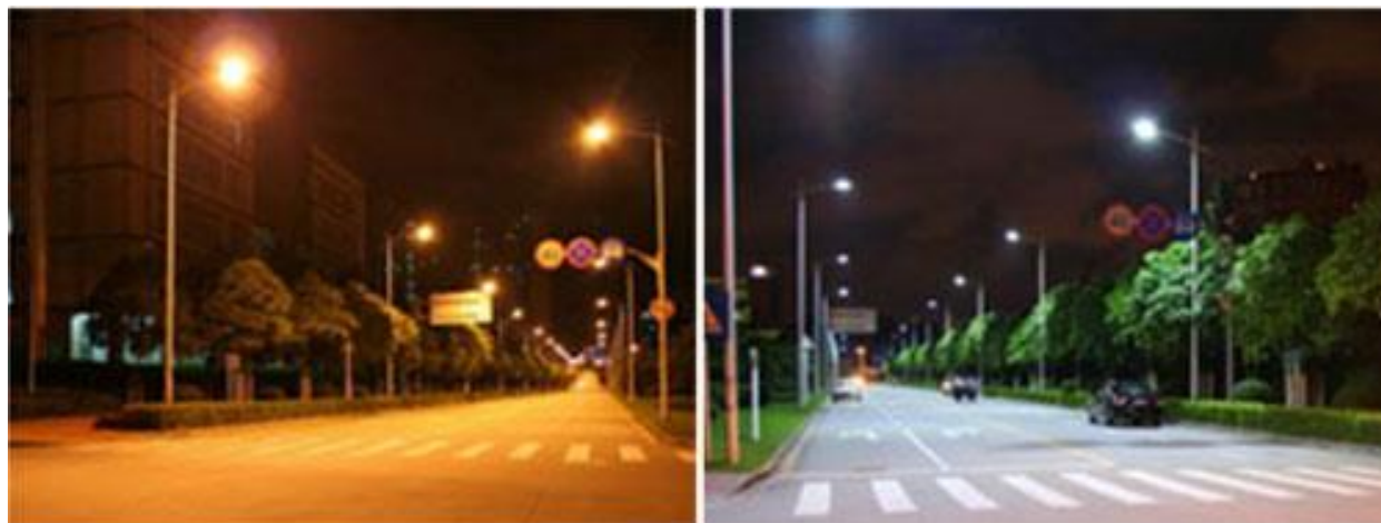
Figure 3-1. Comparison of HPS (left) and LED (right) lighting technologies (Source: ADOT LED Lighting Pilot Study)
