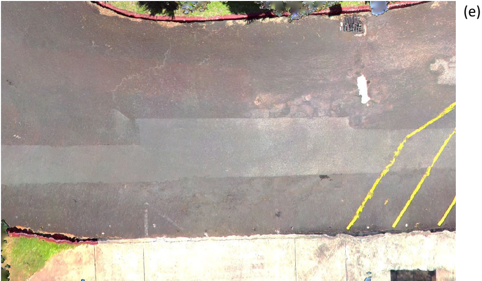
Fig. 21. Examples of georeferenced orthomosaics of roadway.
